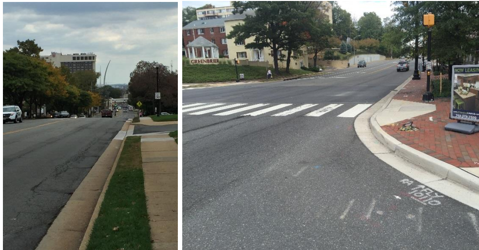
(Left) Example of sidewalk east of Courthouse Road. (Right) Example of sidewalk and crosswalk at S. Greenbrier Street.
