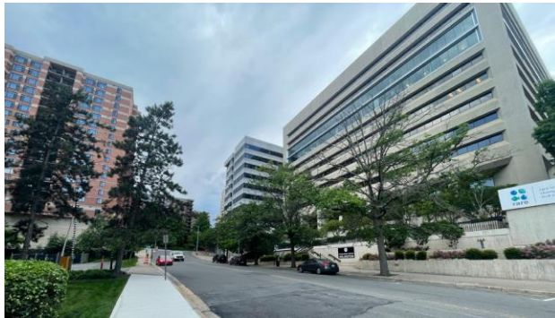
View west along N. 15th Street
