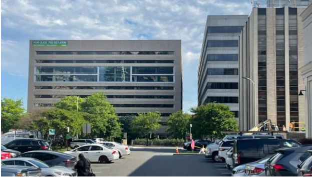
View south from Courthouse Square parking lot
