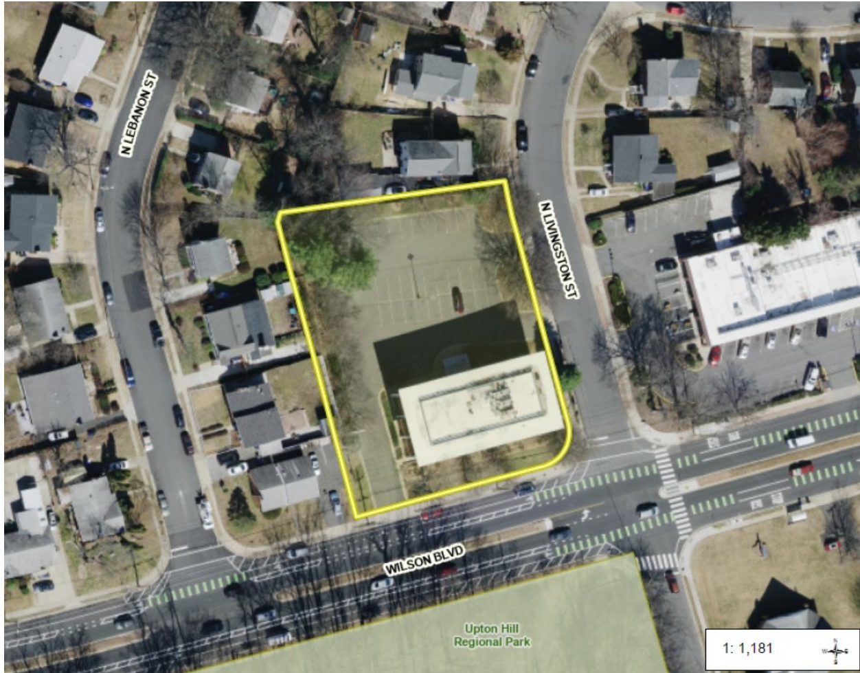
Figure 1: Aerial View (the Property is highlighted in Yellow)
