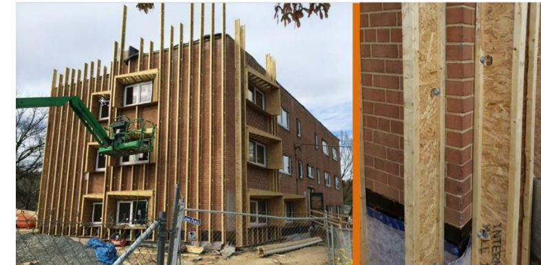
CREATING THE INSULATION CAVITY
