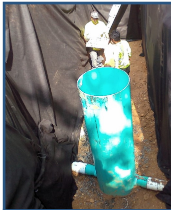
Overflow pipe and perforated underdrain
