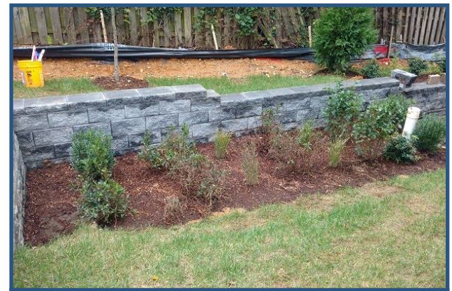
Photo of completed facility showing all plants installed
