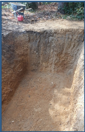
Photo of excavated area
