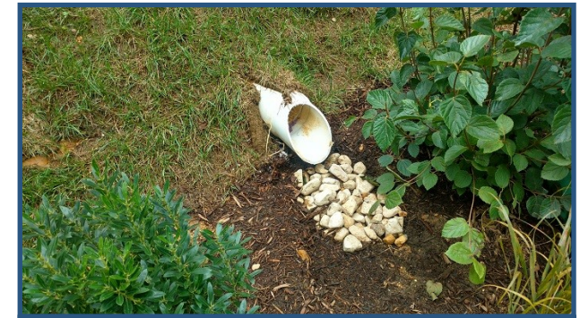
Photos of all inflow to facility (pipe, swale, sheetflow, etc)
