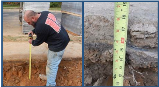
Depth of cut at driveway apron with close up
