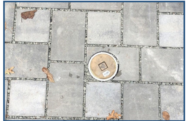
Photo of observation well installed w/ metal cap
