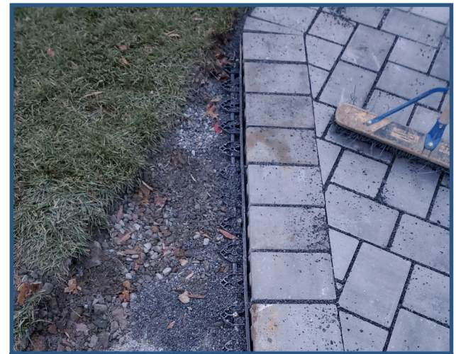
Edge restraints installed
