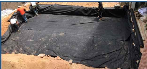
Excavated Subgrade after installing filter fabric
