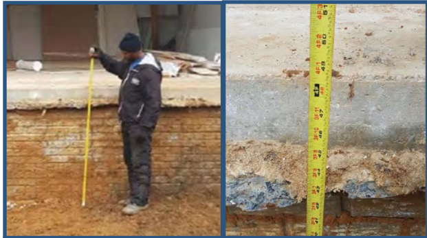
Depth of cut at garage with close up
