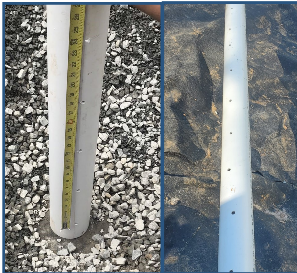
Photos of perforated observation well, perforated underdrain (if required), and storm sewer connection (if required)
