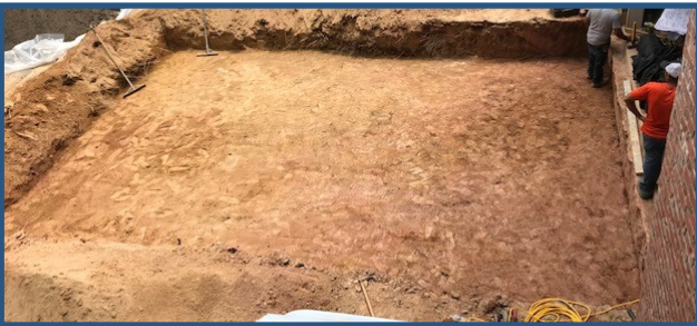
Excavated Subgrade prior to installing filter fabric
