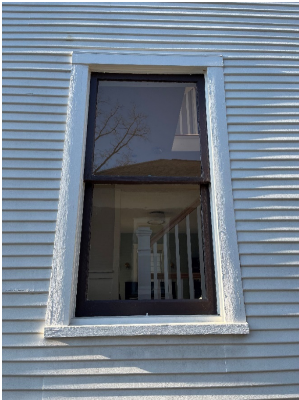
Figure 5 -Existing Double Hung on Historical portion
