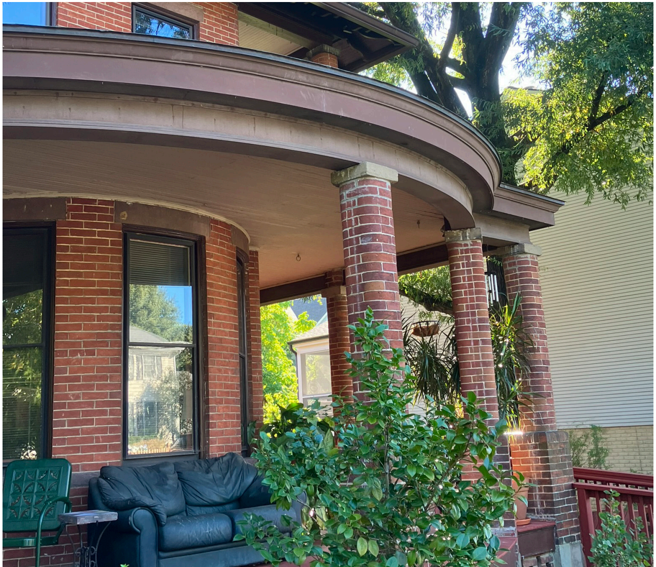
Figure 14: Detail of front porch at 3500 14th St. N. looking southwest. Source: Arlington County Historic Preservation Program, 2022.
