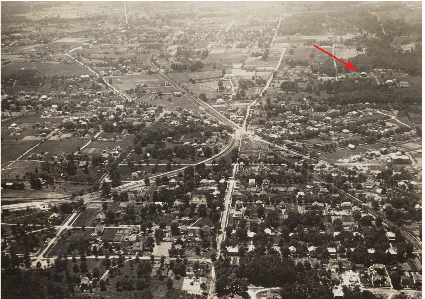
Figure 1: ca. 1921 view of Clarendon looking southeast. The red arrow points to the Anderson House. Source: Library of Congress.
