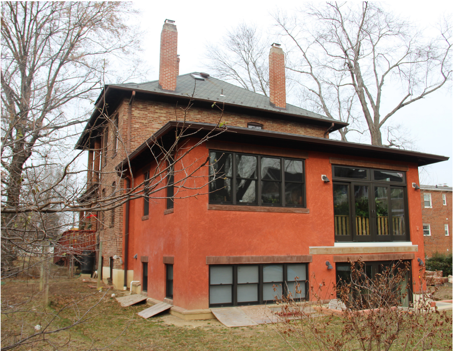
Figure 8: South and west elevations of the home at 3500 14th St. N. looking northeast at 2016 addition. Source: Arlington County Historic Preservation Program, 2018.
