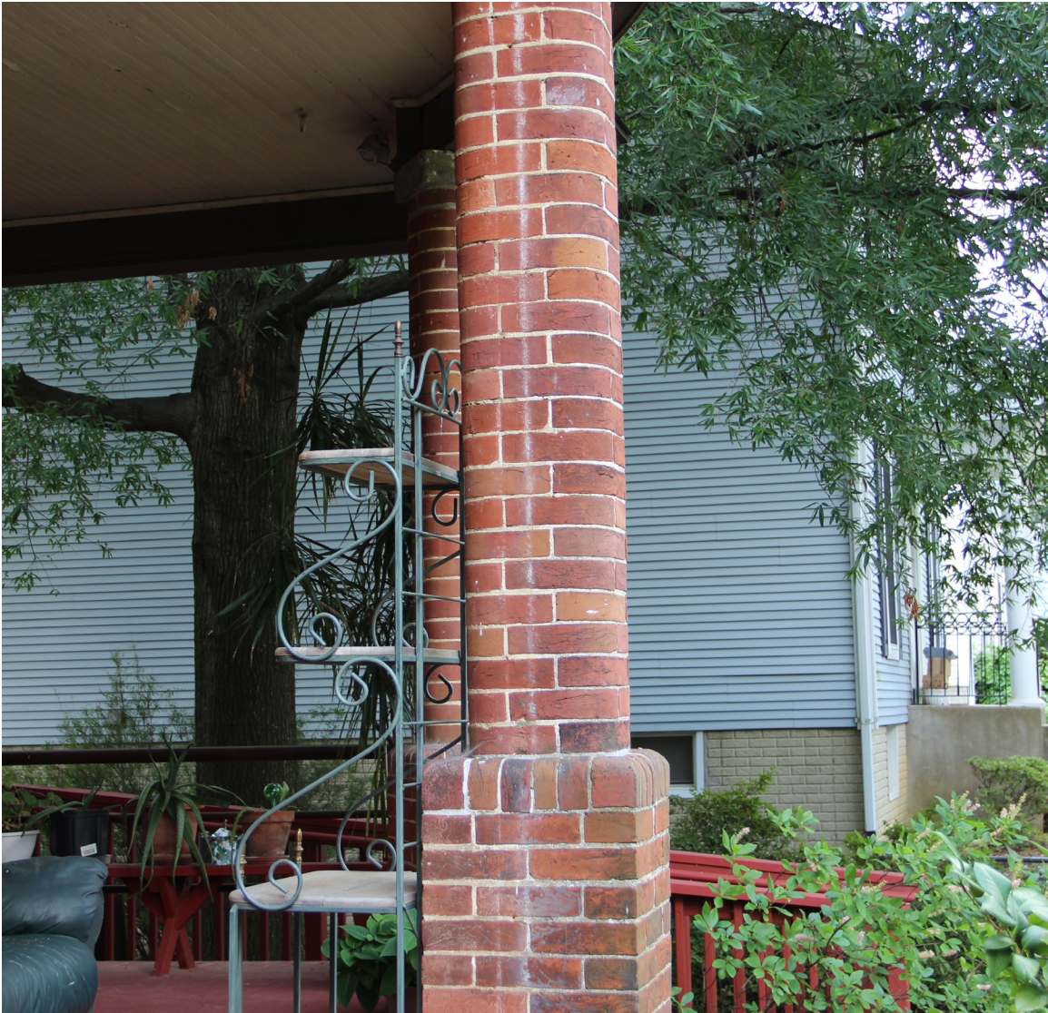
Figure 12: Detail of bullnose radial brick column at 3500 14th St. N. looking southwest. Source: Arlington County Historic Preservation Program, 2016.
