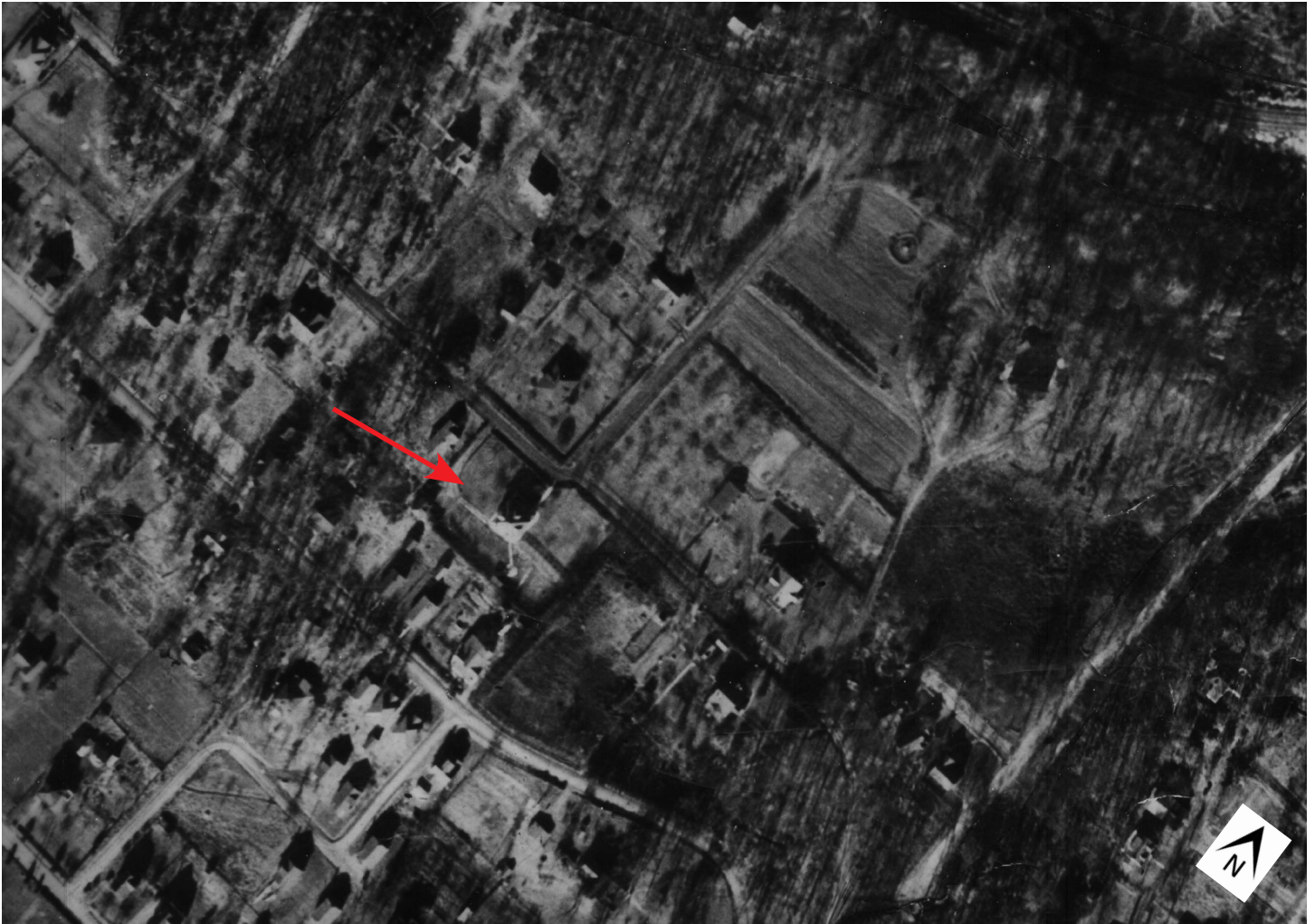
Figure 2: View of the Anderson House, 1934. The red arrow points to the House. Source: Aerial Photographic Map of Arlington County, Virginia . January 11, 1934, Sheet 32, Arlington County GIS.
