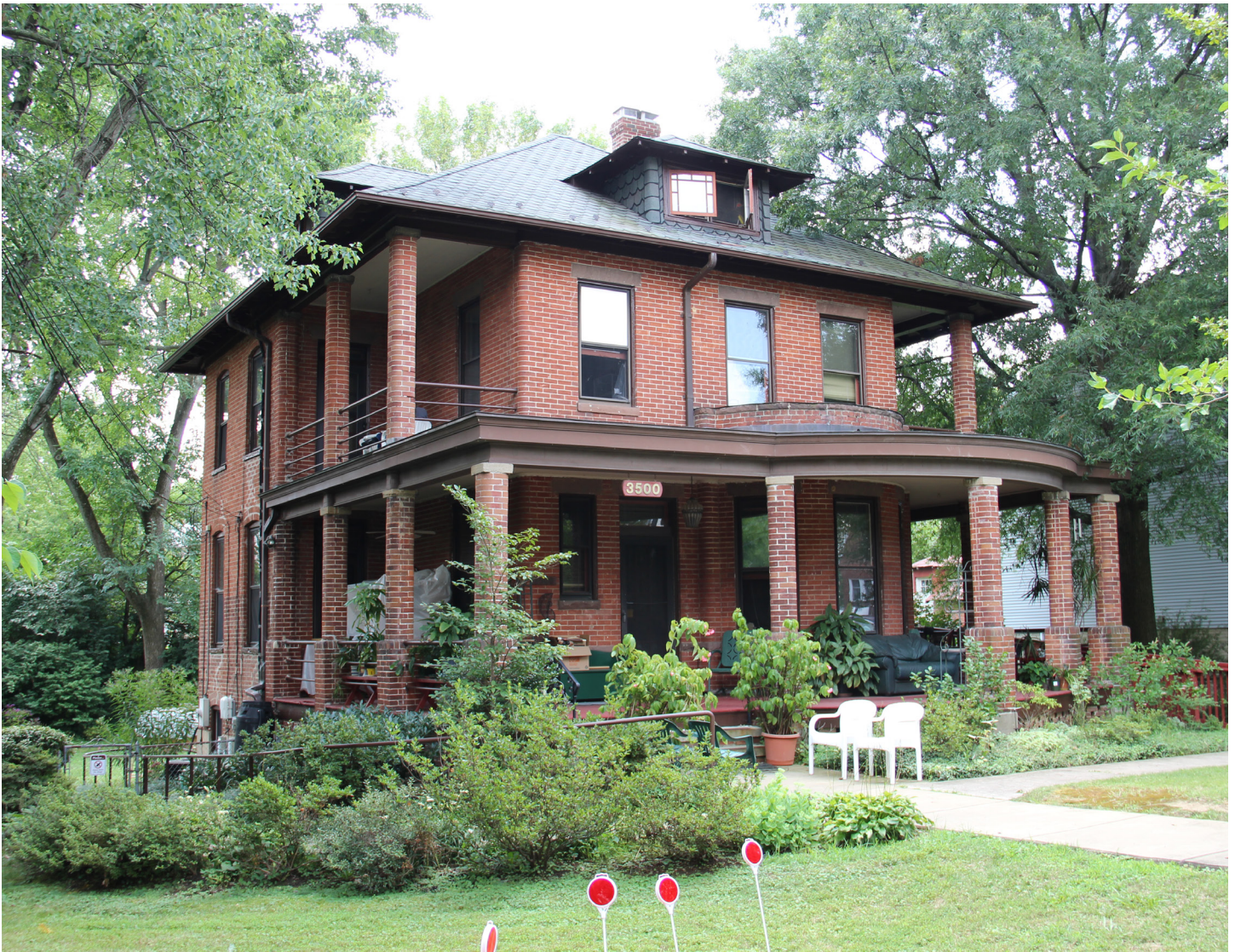
Figure 4: North facade and east elevation of the home at 3500 14th St. N. looking southwest. Source: Arlington County Historic Preservation Program, 2016.
