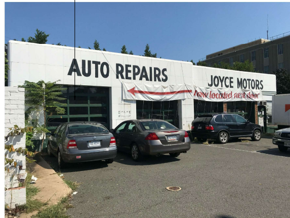
JOYCE MOTORS SOUTH FACADE
