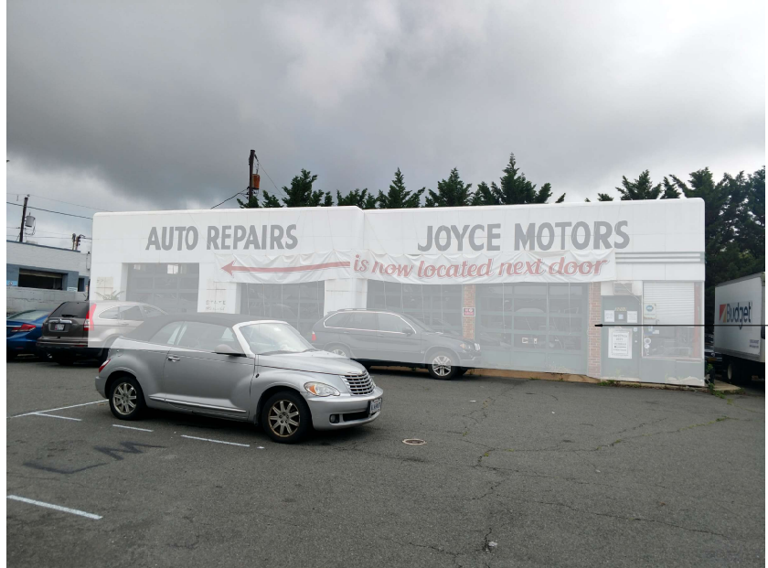
JOYCE MOTORS SOUTH FACADE
