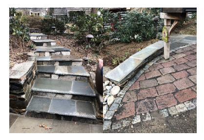
6. Along North Randolph Street, closer to the southwest portion of the property, the applicant installed a granite cobble-stone pull-off area for parking. Originally, the area had been composed of gravel and dirt and was used for the same purpose. To the east of the pull-off area, a stacked stone wall (8-12" in height) composed of the same slate and stone as the new walkway was installed to hold the soil around the region in place. Four LED downlights also were installed in the wall.
