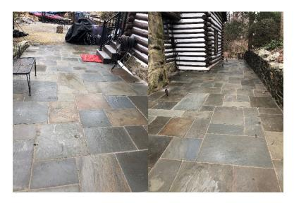
8. Access to the main entrance is granted via two steps; both steps were narrow and did not allow for those entering the house to stand on them while opening the door. The applicant has since extended the tread of the two steps with slate matching the original stairs. The area outlined in red is the earlier stair.
