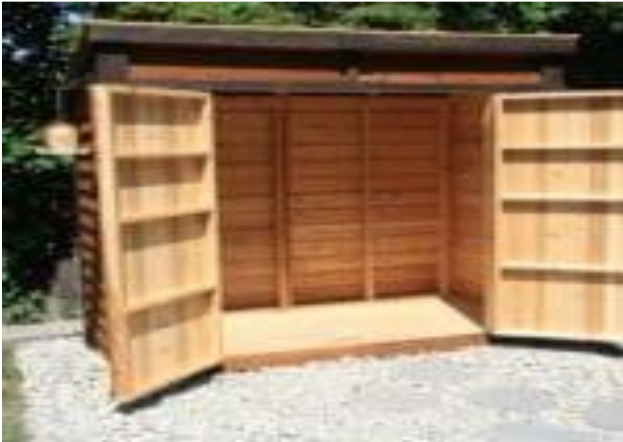
Proposed Garden Shed with doors open. Dimensions are 8 feet wide like garden beds, 6 feet deep and 7.25 Feet at the front with a sloped roof 6.6 feet at the back.
