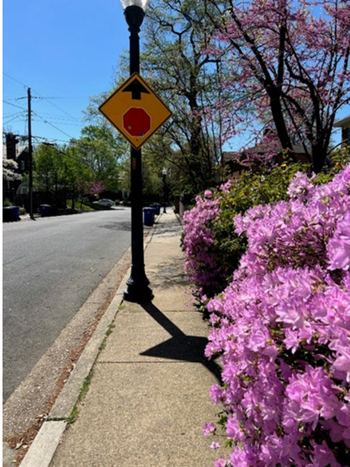
Sidewalk on the west side obstructed by streetlights
