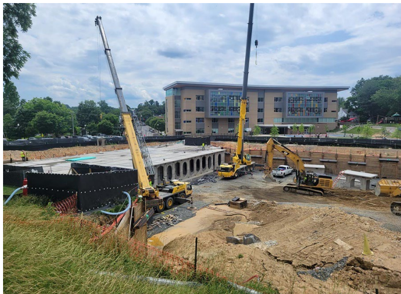
Work on the Cardinal Elementary Stormwater Vault
