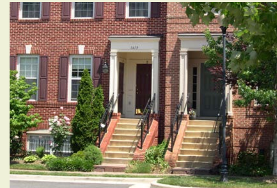
Buildings with English basements may have first floors above grade, as illustrated above. Urban and 9th Road Residential frontage types may include English basements.
