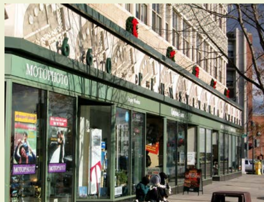
660 Pennsylvania Ave. SE, Washington, DC
