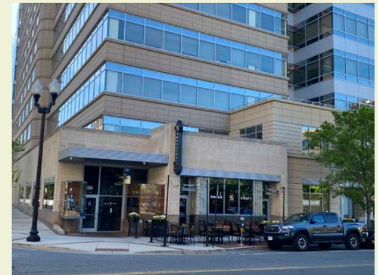
1041 North Highland Street
