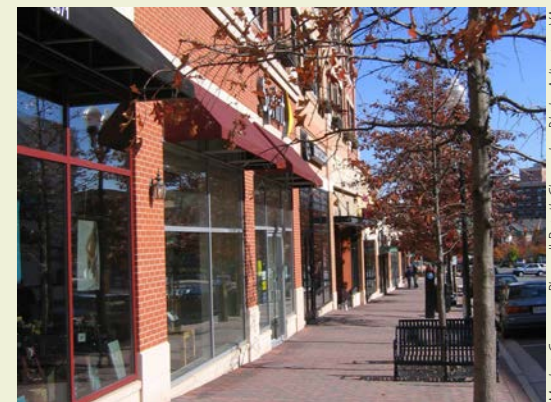
Marker Common Phase II Retail, Clarendon Blvd., Arlington, VA
