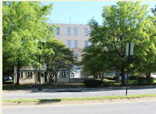
County and Verizon Properties
