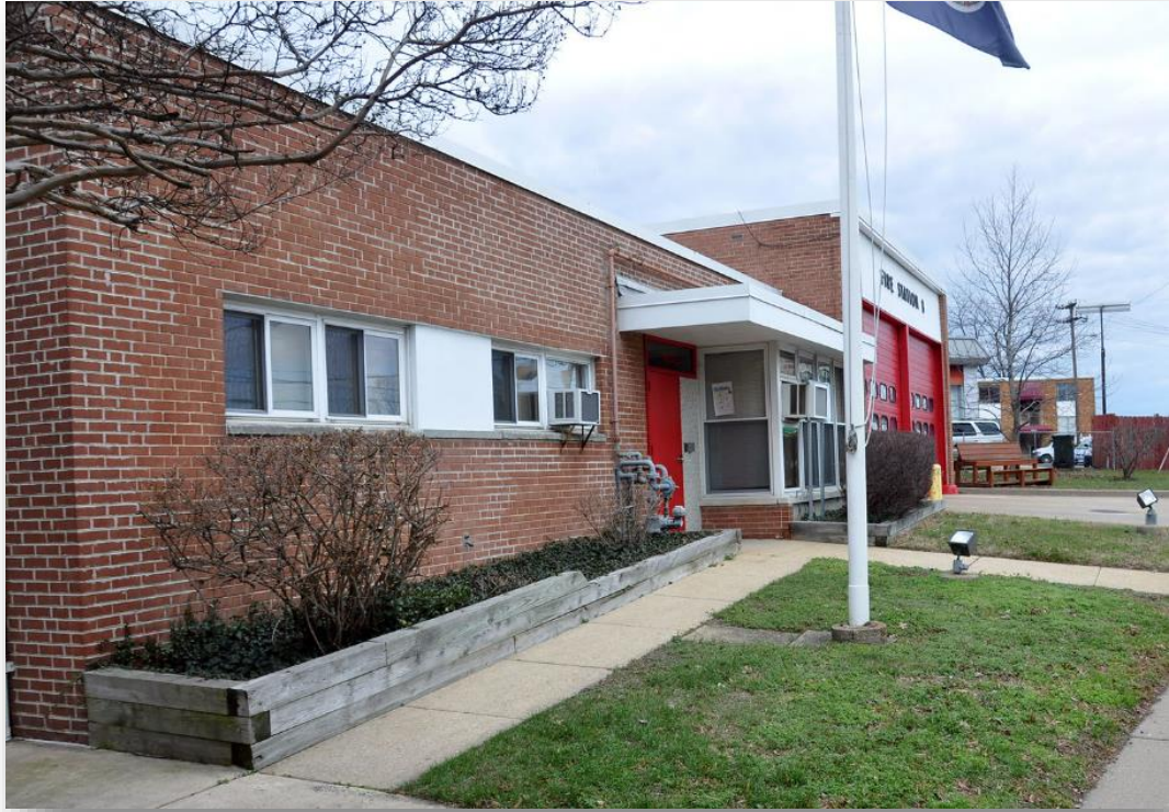
Photo credit: Fire Station 8 Task Force, January 2016
