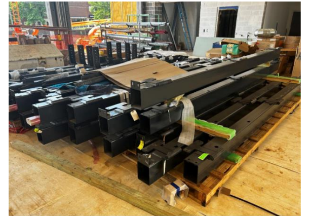
Four-fold doors to be installed
