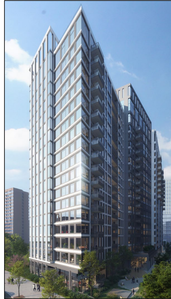
Richmond Highway Frontage
