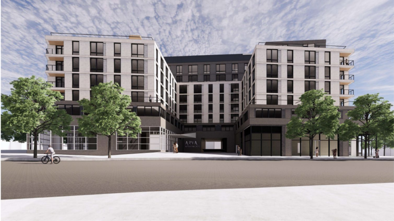
CONTEXT VIEW - PERSHING DRIVE - LOOKING INTO THRU-BLOCK ACCESS Figure 7---Courtesy Applicant
