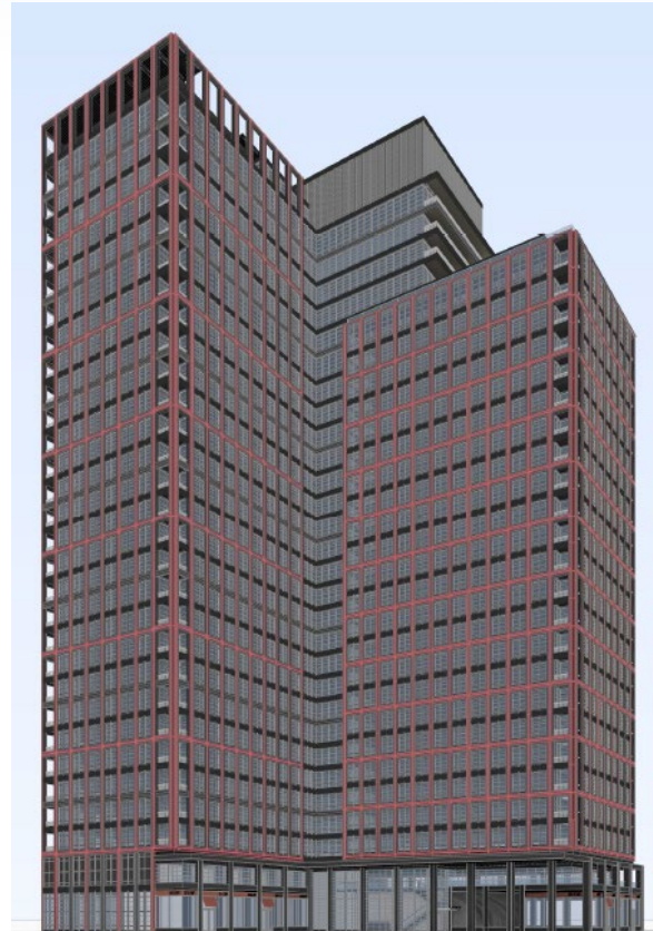
Original Building Design
