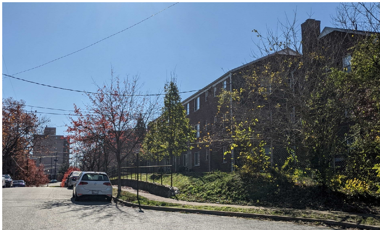
3. NORTH ODE ST. LOOKING SOUTHEAST
