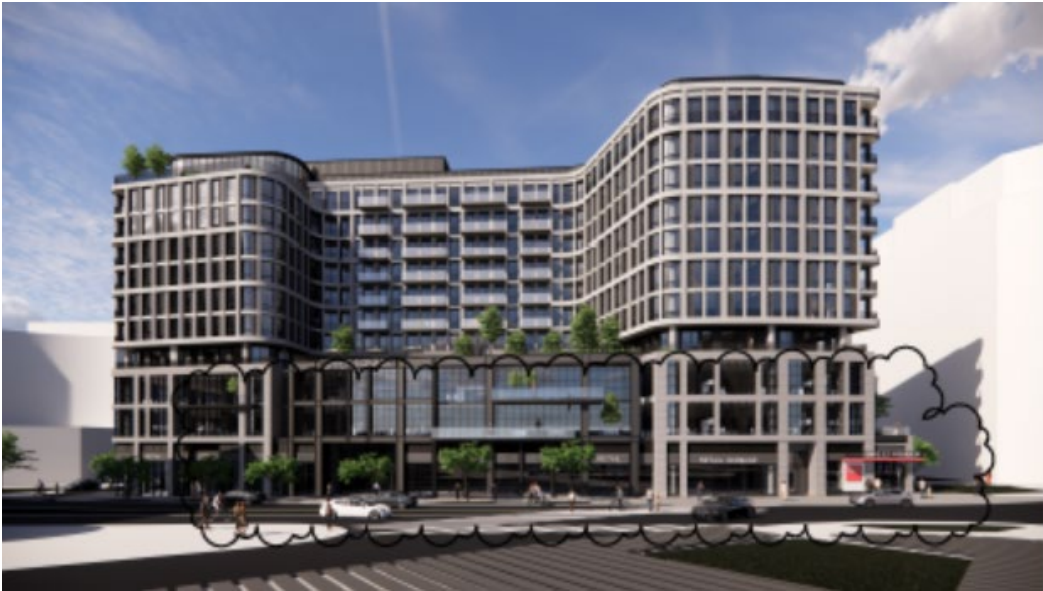
Wash Blvd (N) Facade
