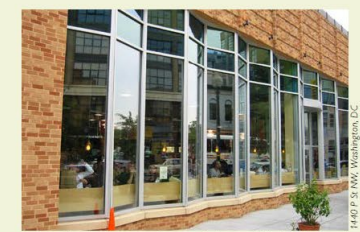
Interesting designs, sturdy materials, careful detailing, and ample transparency are encouraged along Clarendon's "Main Street" frontages.
