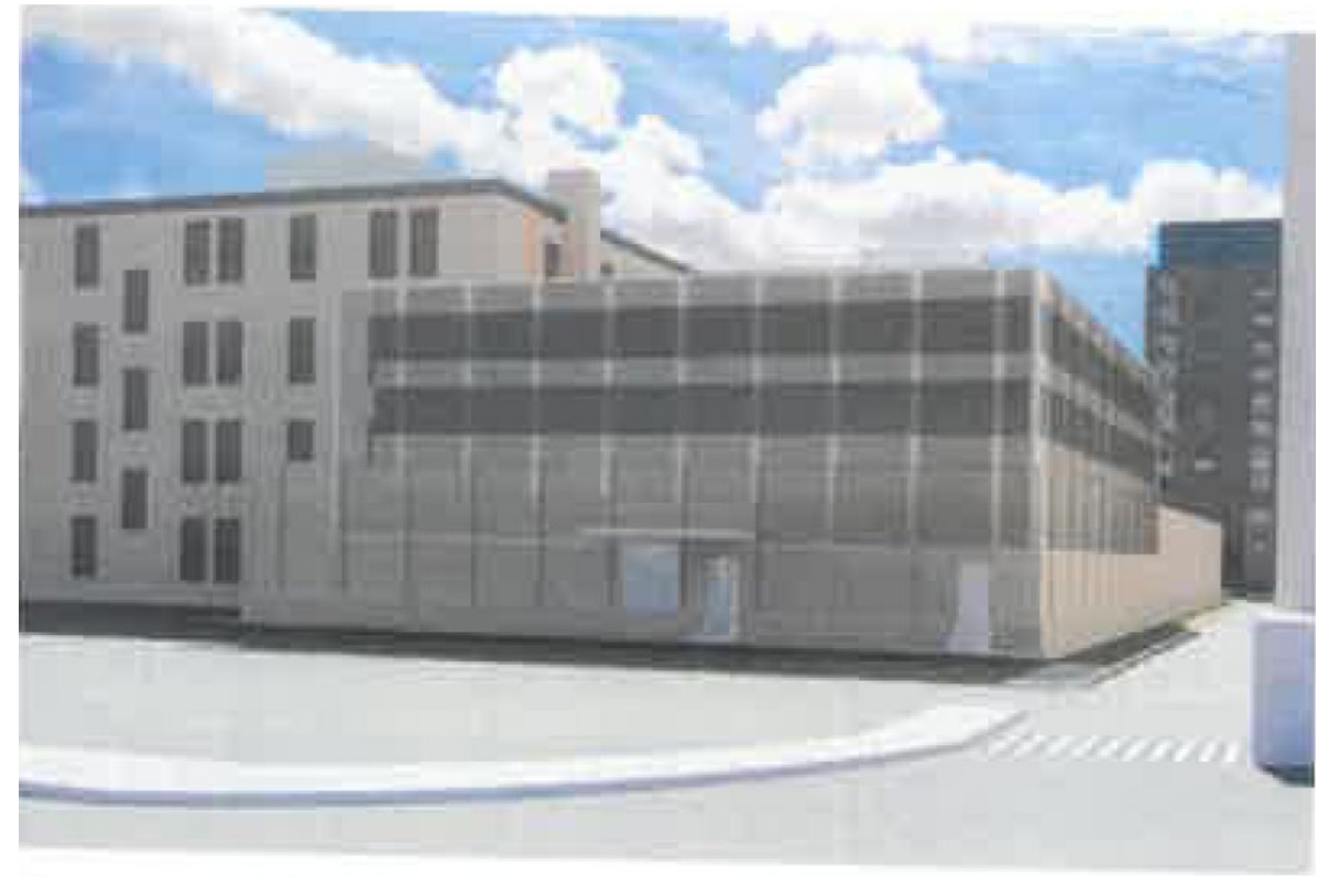
/view from N. Hudson Street
