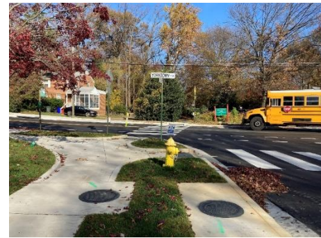
Quick build project at Yorktown Blvd & George Mason Dr
