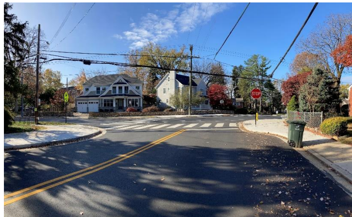
Quick build project at 26th St N & Harrison St
