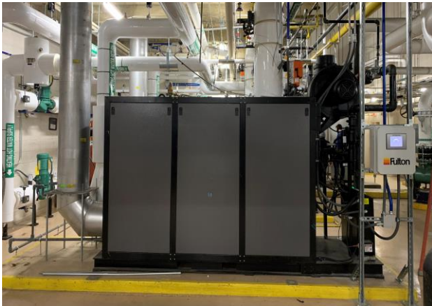
Justice Center Boiler Replacement
