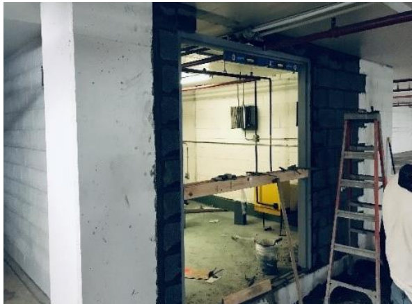
CSI - ECC Emergency Generator in BGC
