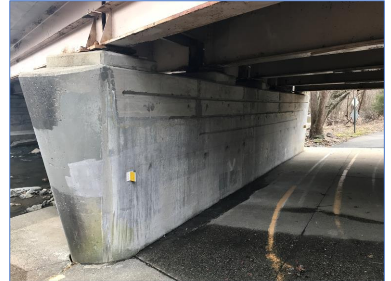
After concrete repairs
