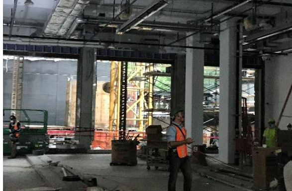
Fire Station #10 Apparatus Bay
