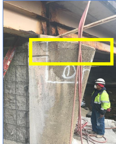
Before concrete repairs
