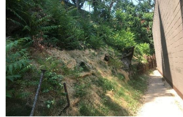
Retaining Wall for Eads Warehouse
