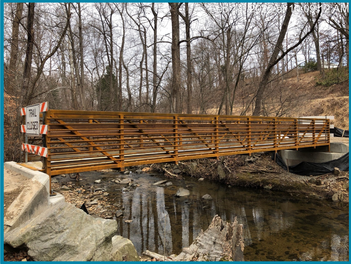
Glencarlyn Bridge (bridge installed February 2022)
