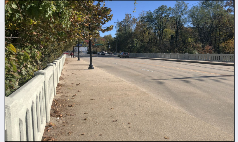
Columbia Pike - Four Mile Run Bridge ($0.6m) Completed fall 2021
