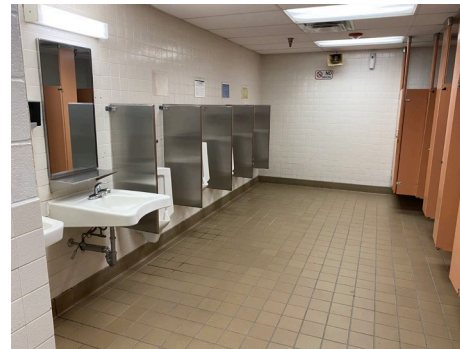
WSS Restroom Refresh $390K, 50% complete
