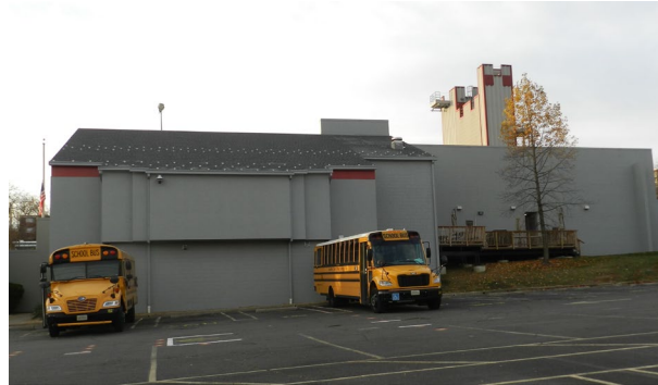
Fire Training Academy Façade Repair
