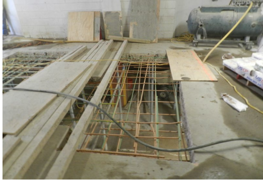
CSW Garage Repair $495K, 95% Complete
