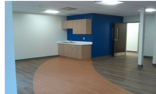
Arlington Childcare Center Renovation
