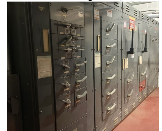
CSW Electrical Switchgear Replacement
