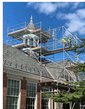
Fairlington Community Center Cupola Repair $170k, 80% Complete
