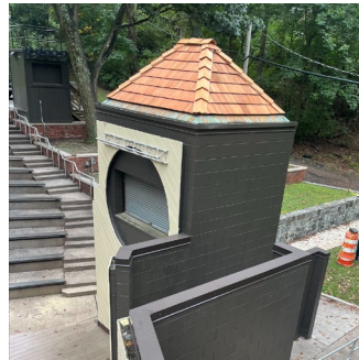
Lubber Run Amphitheatre Roof and Retaining Wall Repair
