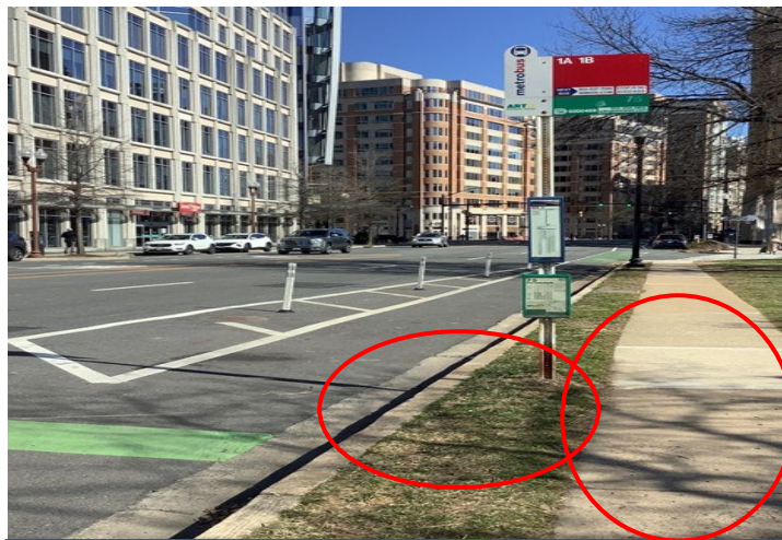
Compliance = regrade sidewalk and install pad to curb
