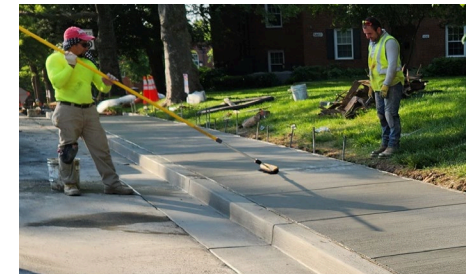
Crews installing new sidewalk
