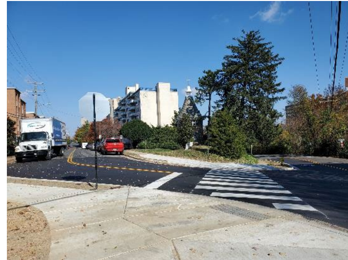
Arlington Ridge / Lynn St. Improvements (total cost $1.2m) Almost Completed
