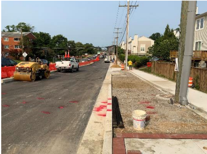
Columbia Pike – Segment F (total cost $45.1m) Completion Anticipated Summer 2025
