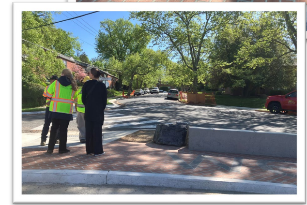
(project in construction)
