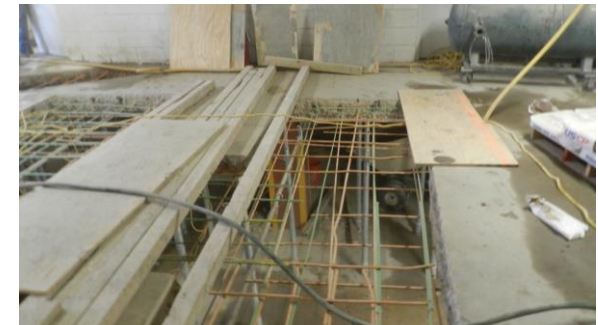
Court Square West Garage Repairs
