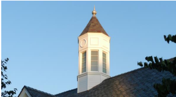
Fairlington Community Center Cupola Repair
