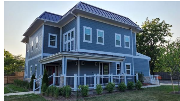
1212 S. Irving Group Home Construction and Solar Installation
