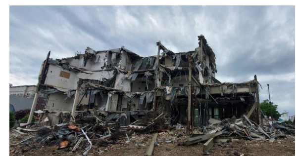
3108 Columbia Pike Demolition
