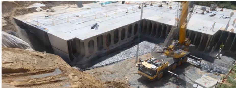
Cardinal School Detention Vault – Construction
