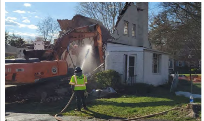
Demolition of 4437 18th St. N
