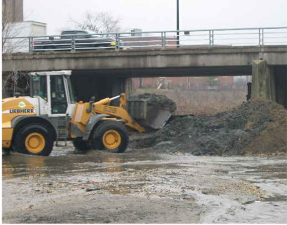
Four Mile Run Dredging
