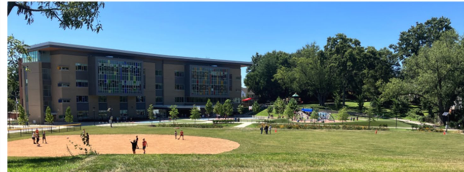
Cardinal School Detention Vault – Complete
