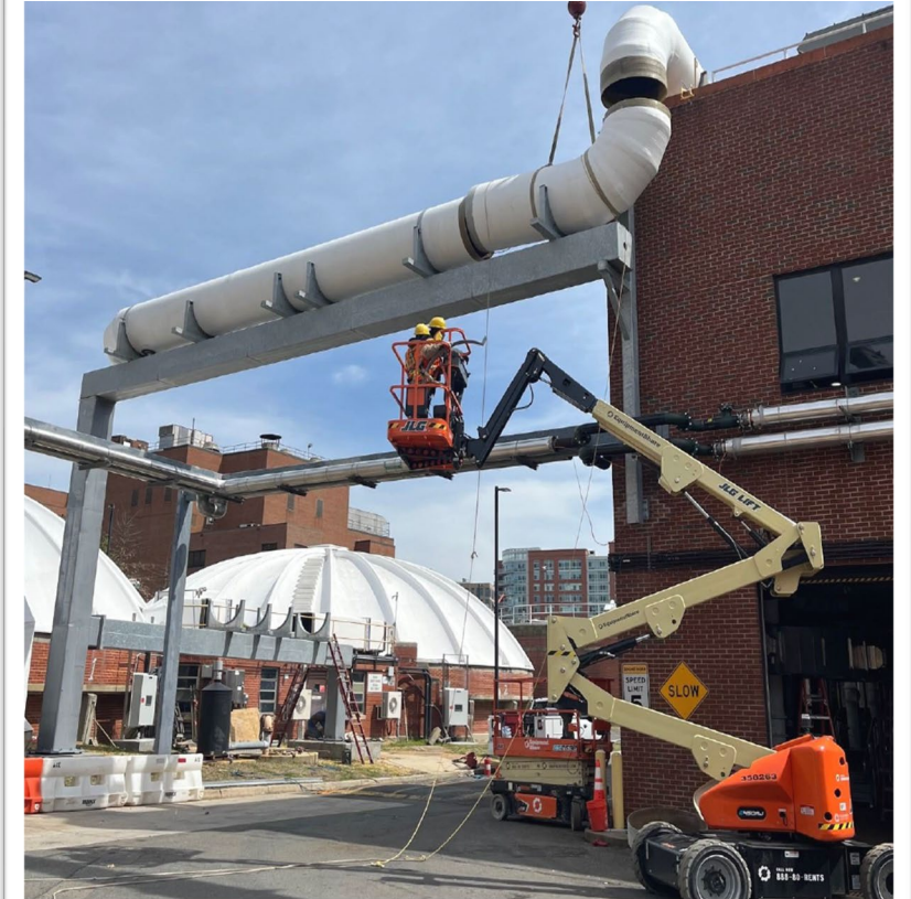
Preliminary Treatment Building Bar Screens/Odor Control Upgrades
