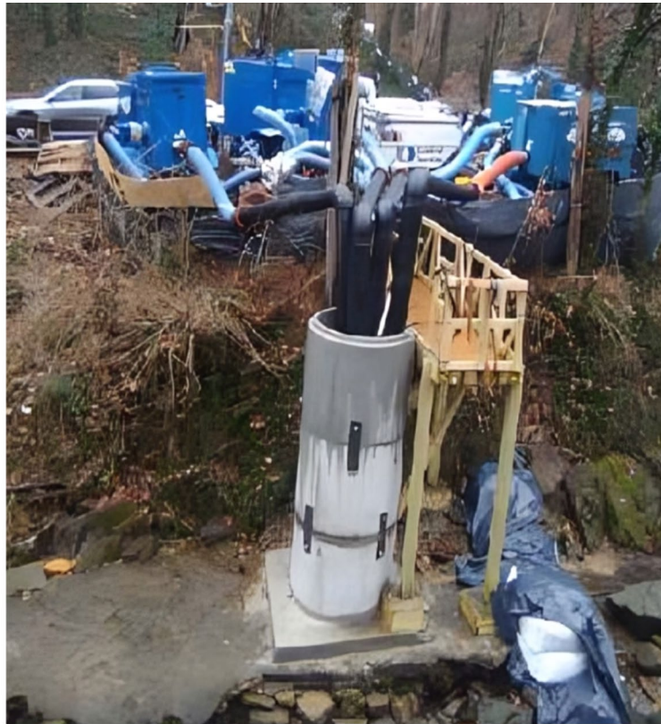
33" Spout Run Deep Sewer Relining and Rehabilitation
