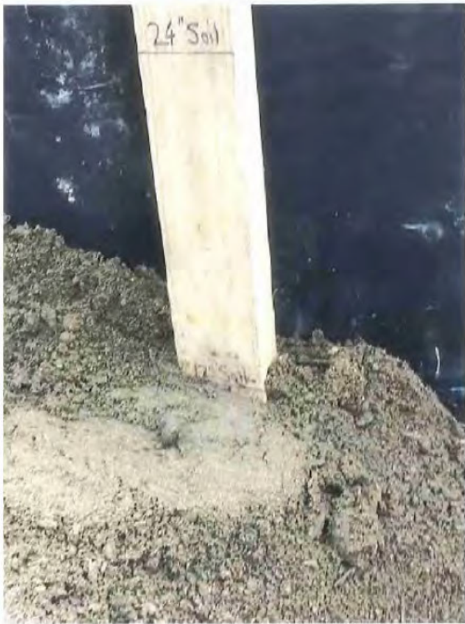
First 2 feet of soil media installed in Tree Filter #2
