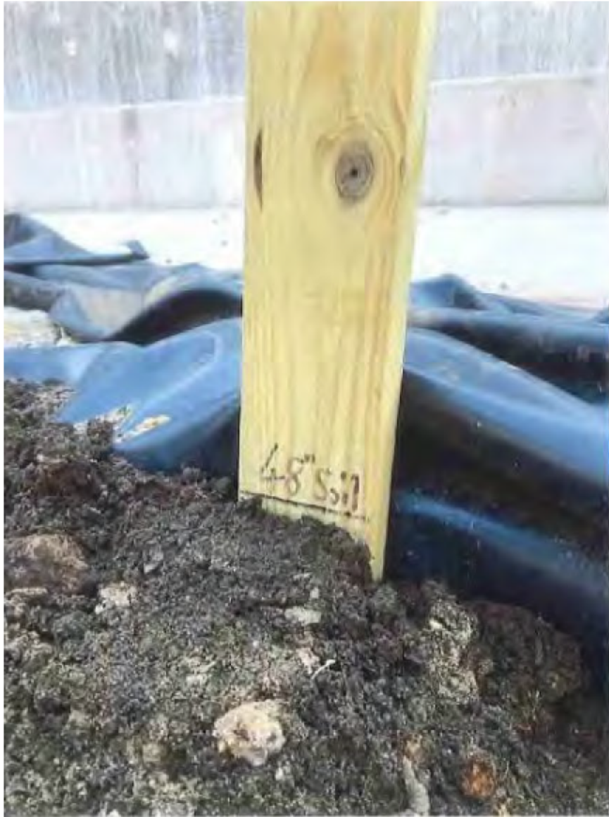
4 feet of soil media installed in Tree Filter #2
