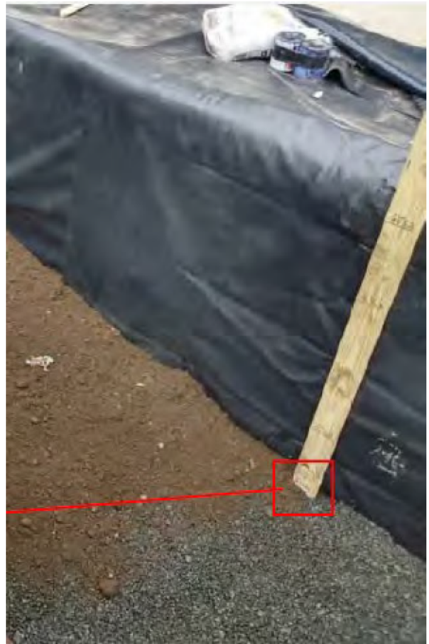
#8 stone installed in Tree Filter #2, 3"
