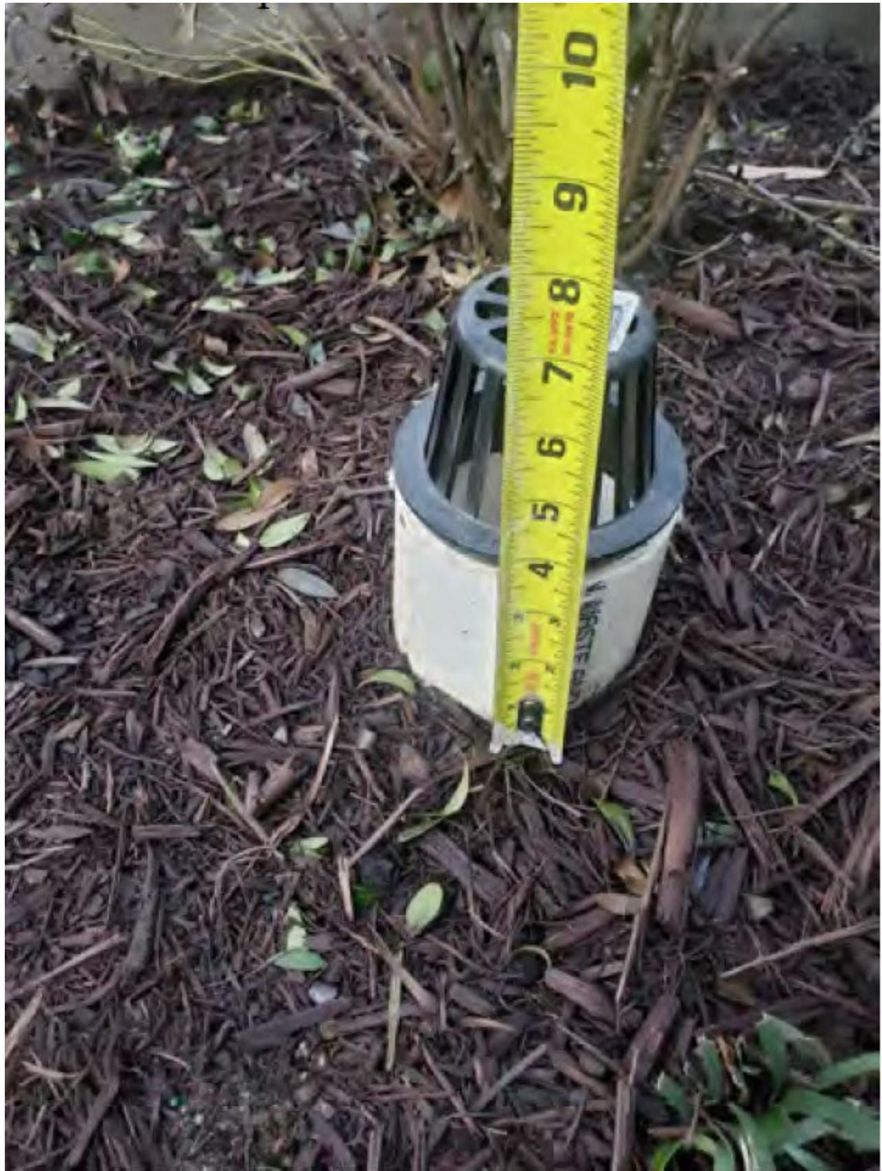
Tree Filter #2: Top of mulch to crest of overflow pipe, Ponding Depth = 4"
