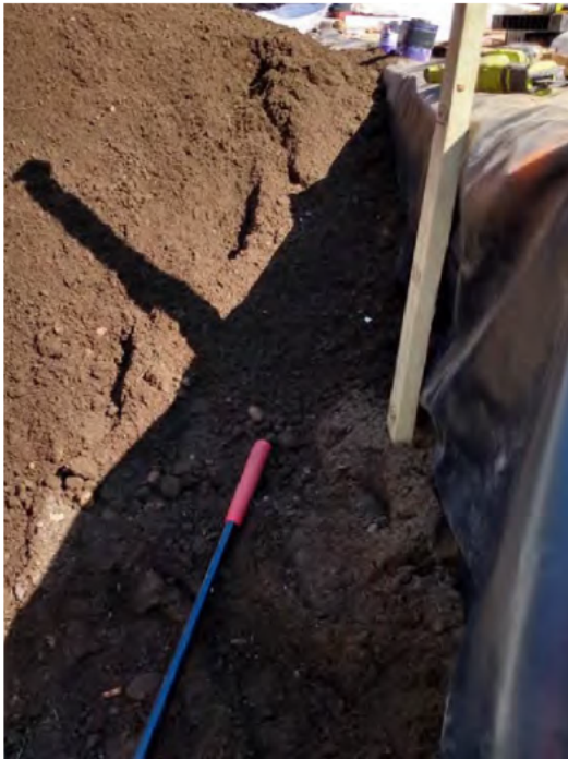
4 feet of soil media installed in Tree Filter #3
