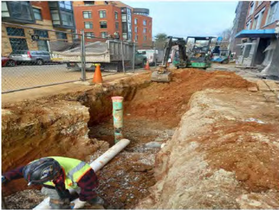
Photo 1: Bioretention # 2 Excavation process
