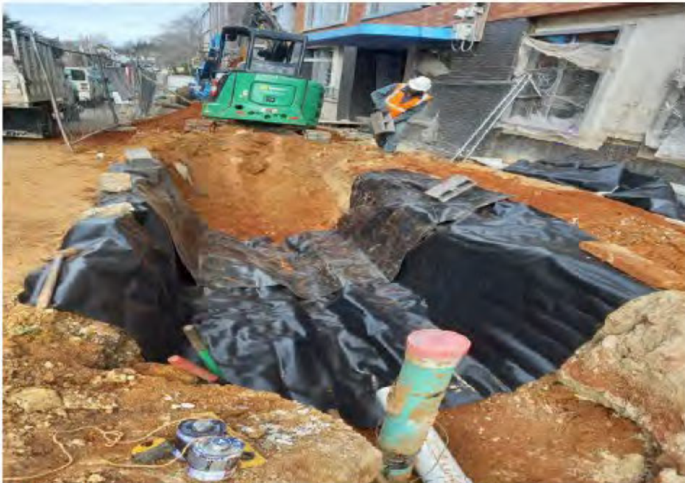
Photo 2: Bioretention # 2 Impermeable liner material laid on sides of the facility
