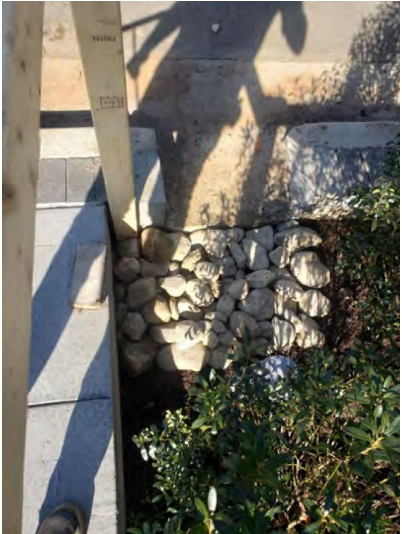
Tree Filter #2: Curb Cut inflow with splash rocks installed
