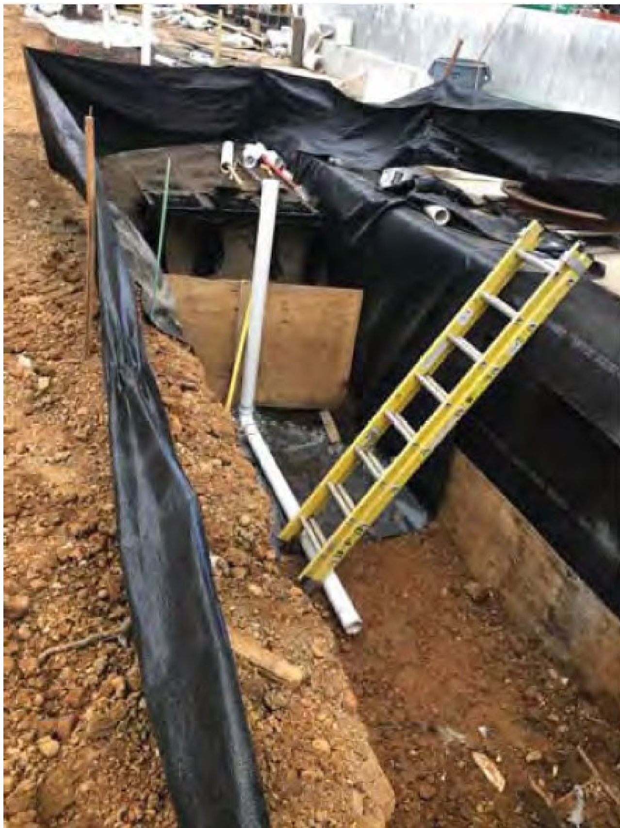
Tree Filter #1: Excavation and installation of impermeable liner
