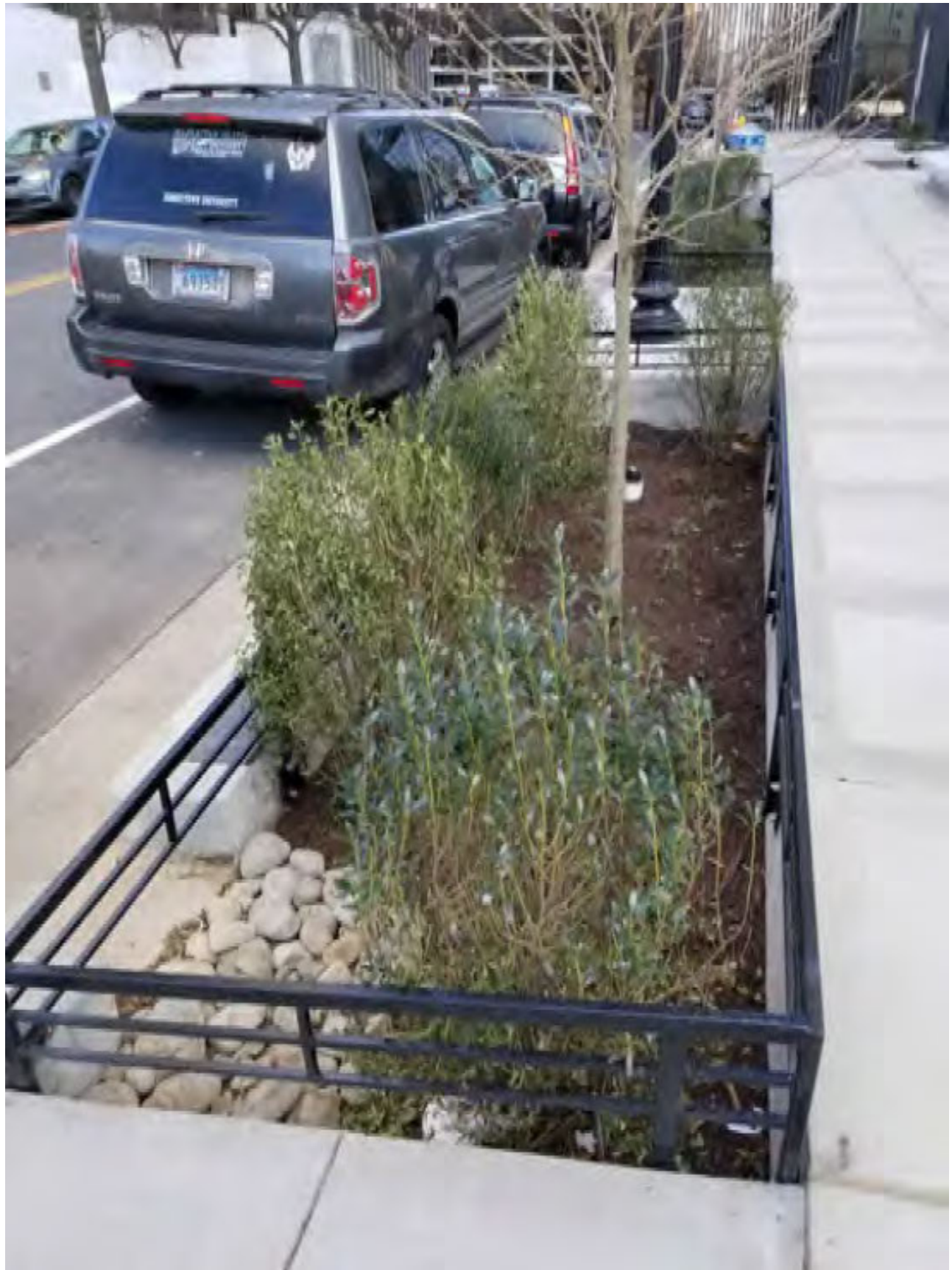
Tree Filter #3: Overall completed tree filter facility with plants, mulch, and splash rocks installed.
