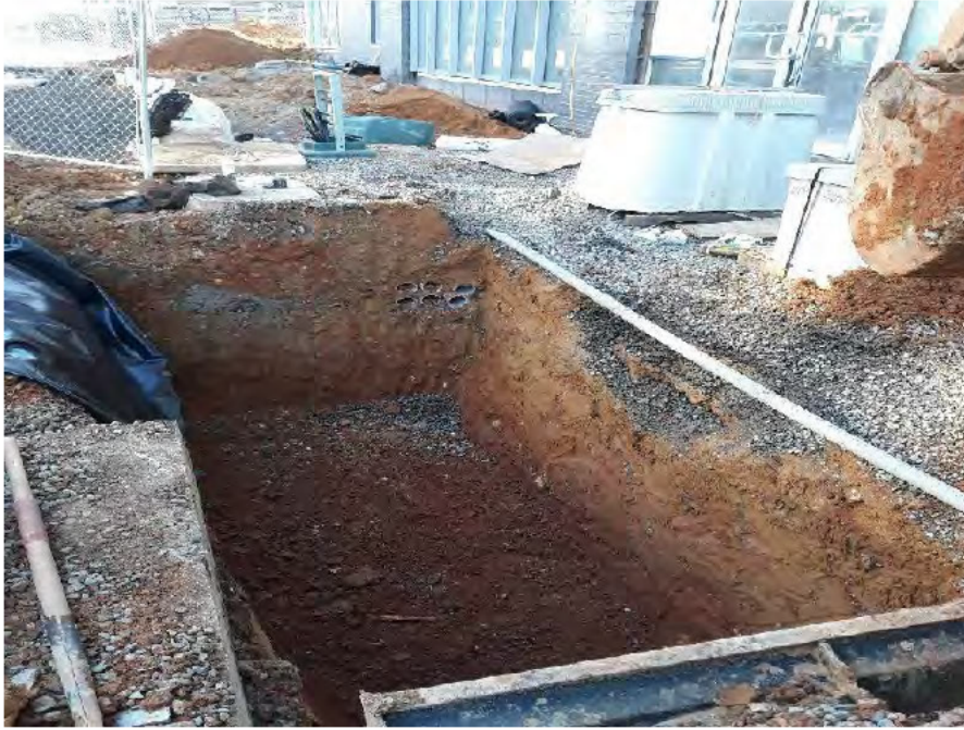
Tree Filter #3 excavation
