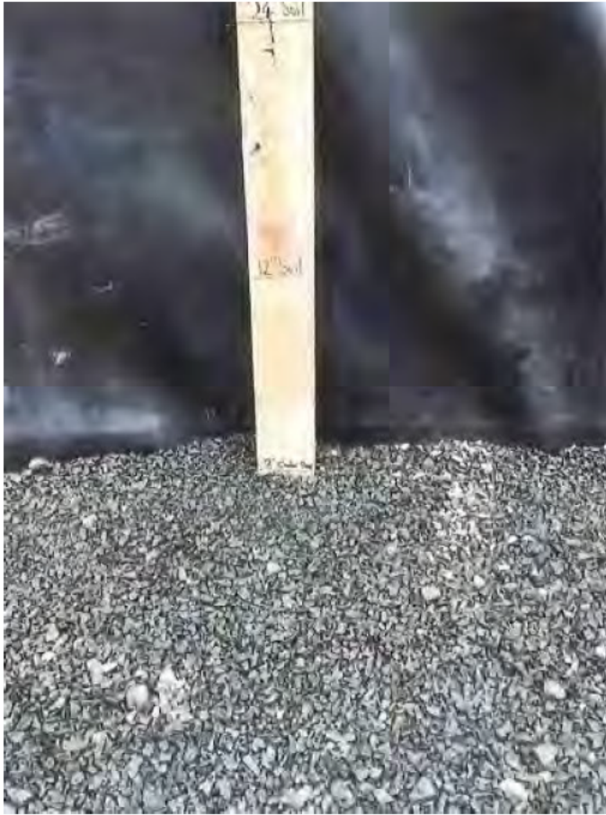
#8 stone installed in Tree Filter #3, 3"
