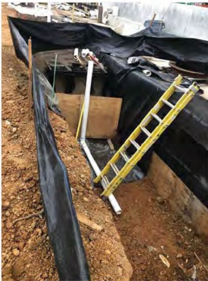
Impermeable liner and underdrain installation
