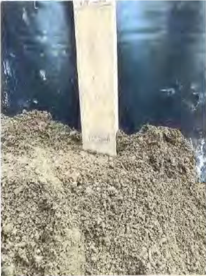
First 2 feet of soil media installed
