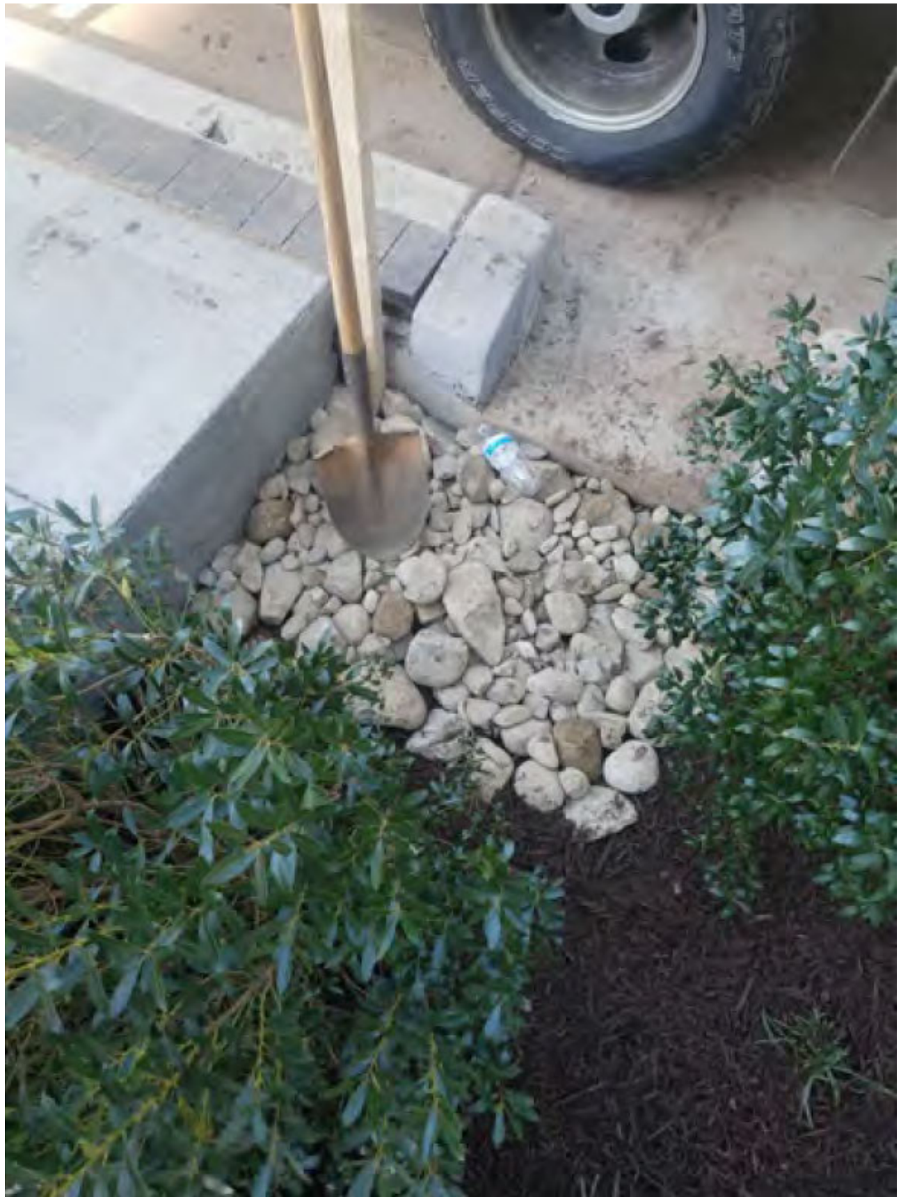
Tree Filter #3: Curb Cut inflow with splash rocks installed
