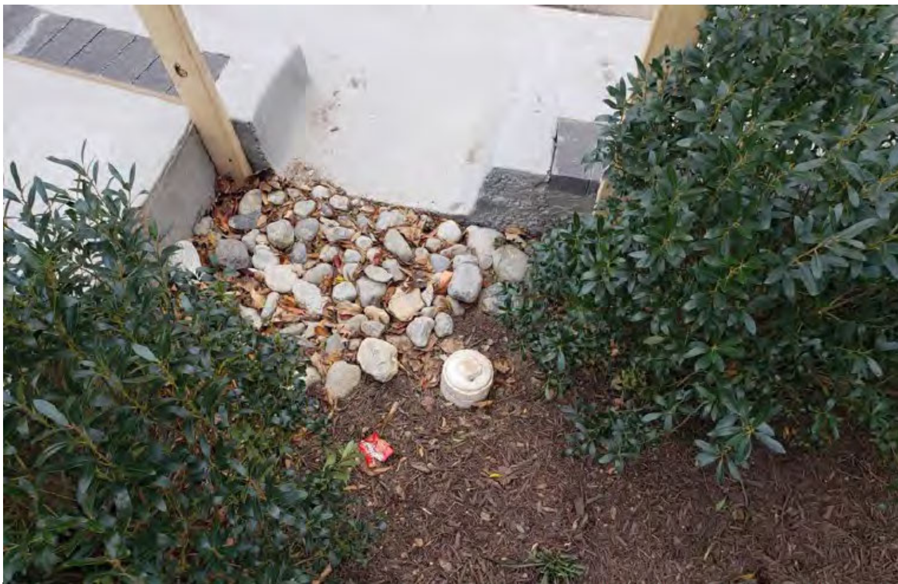
Tree Filter #1: Curb Cut inflow with splash rocks installed
