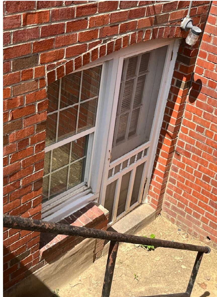
/ BUILDING 32 EXISTING REAR ENTRY DOORS
