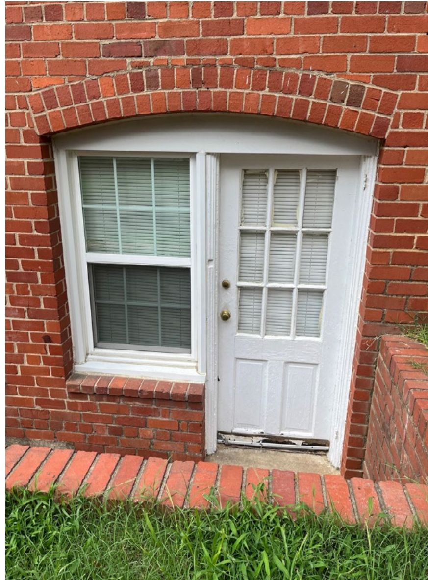
/ BUILDING 30 EXISTING REAR ENTRY DOORS
