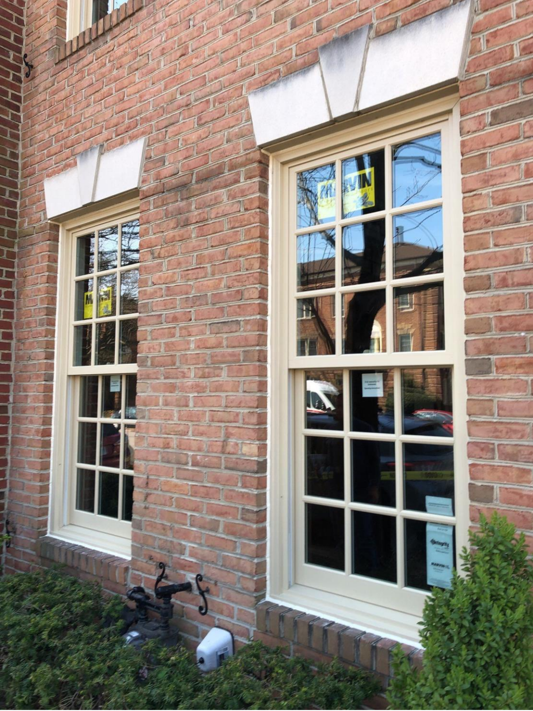
Pictures of existing windows.
