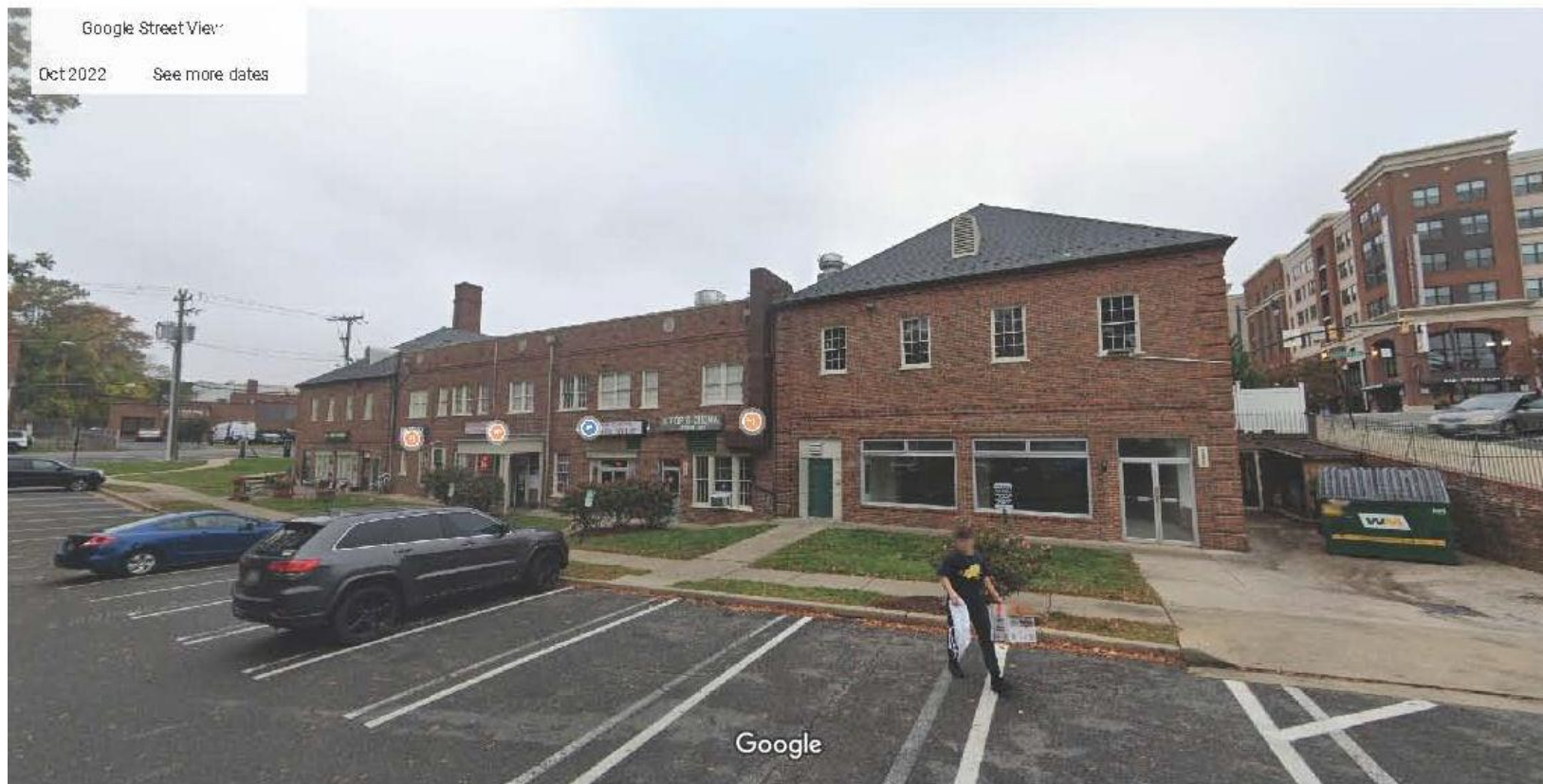
Shopping Center - Rear elevation - View of area of proposed work
