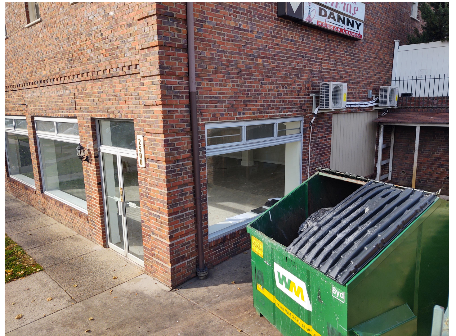
Celtic House Rear Elevation corner detail at area of proposed work
