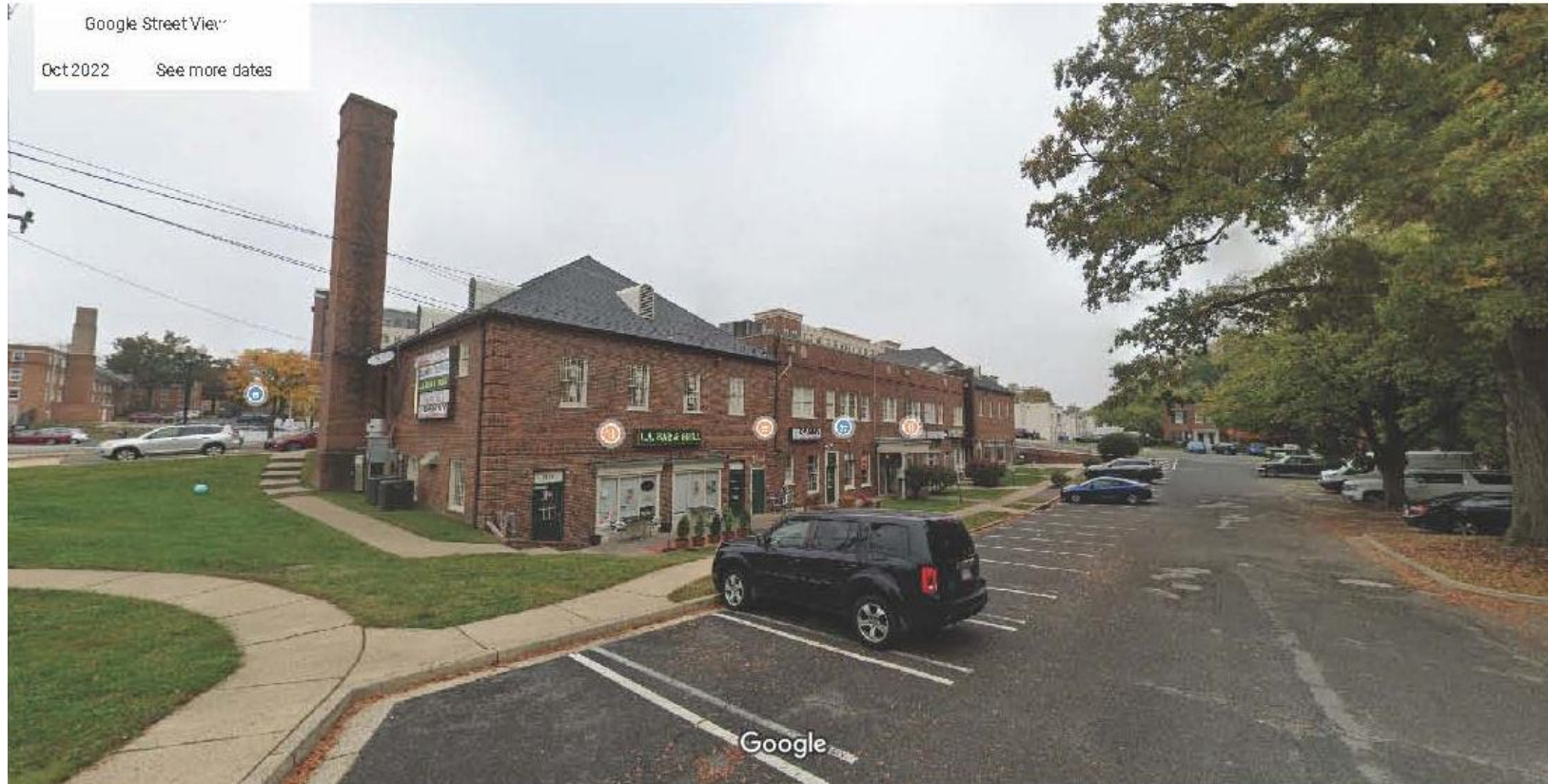
Shopping Center - Rear elevation - View at other end of building
