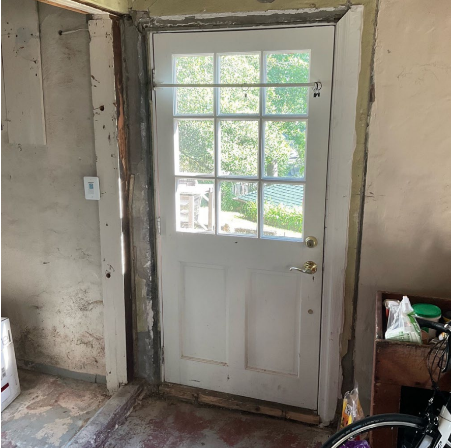
Existing Basement door circa 1984
