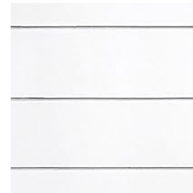
WOOD LAP SIDING, REPAIRED / REPLACED IN PLACE
