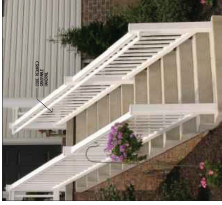
5 EXAMPLE OF GRASPABLE HANDRAIL NTS
