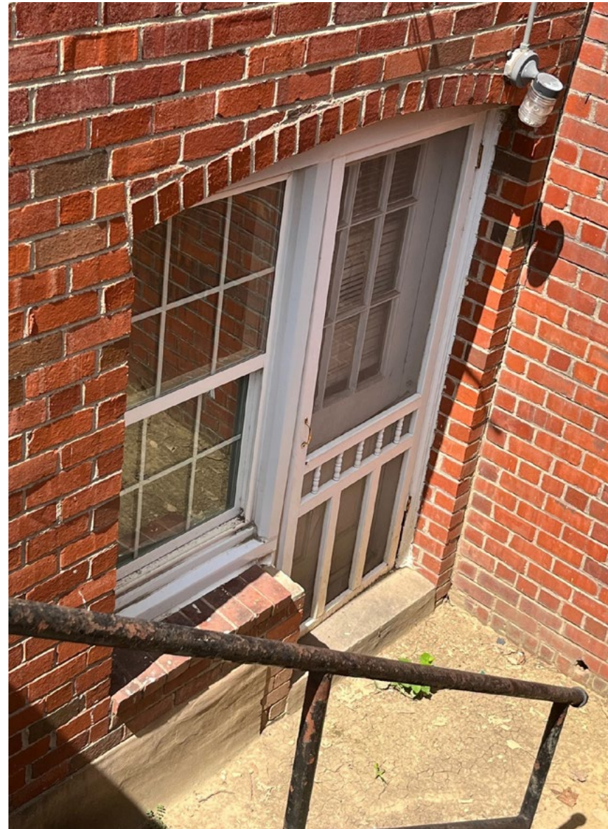
/ BUILDING 32 EXISTING REAR ENTRY DOORS
