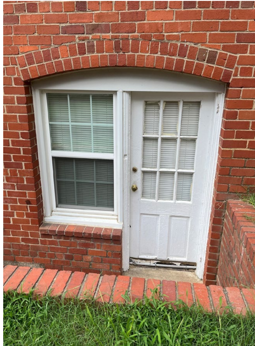
/ BUILDING 30 EXISTING REAR ENTRY DOORS
