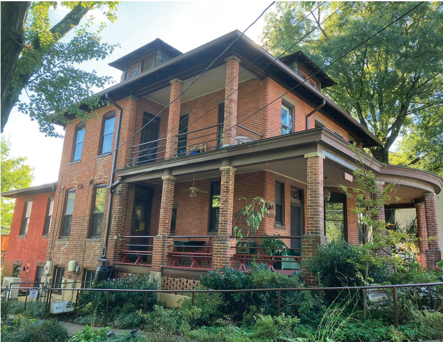
Figure 6: East elevation of the home at 3500 14th St. N. looking southeast with 2016 addition visible in rear. Source: Arlington County Historic Preservation Program, 2022.
