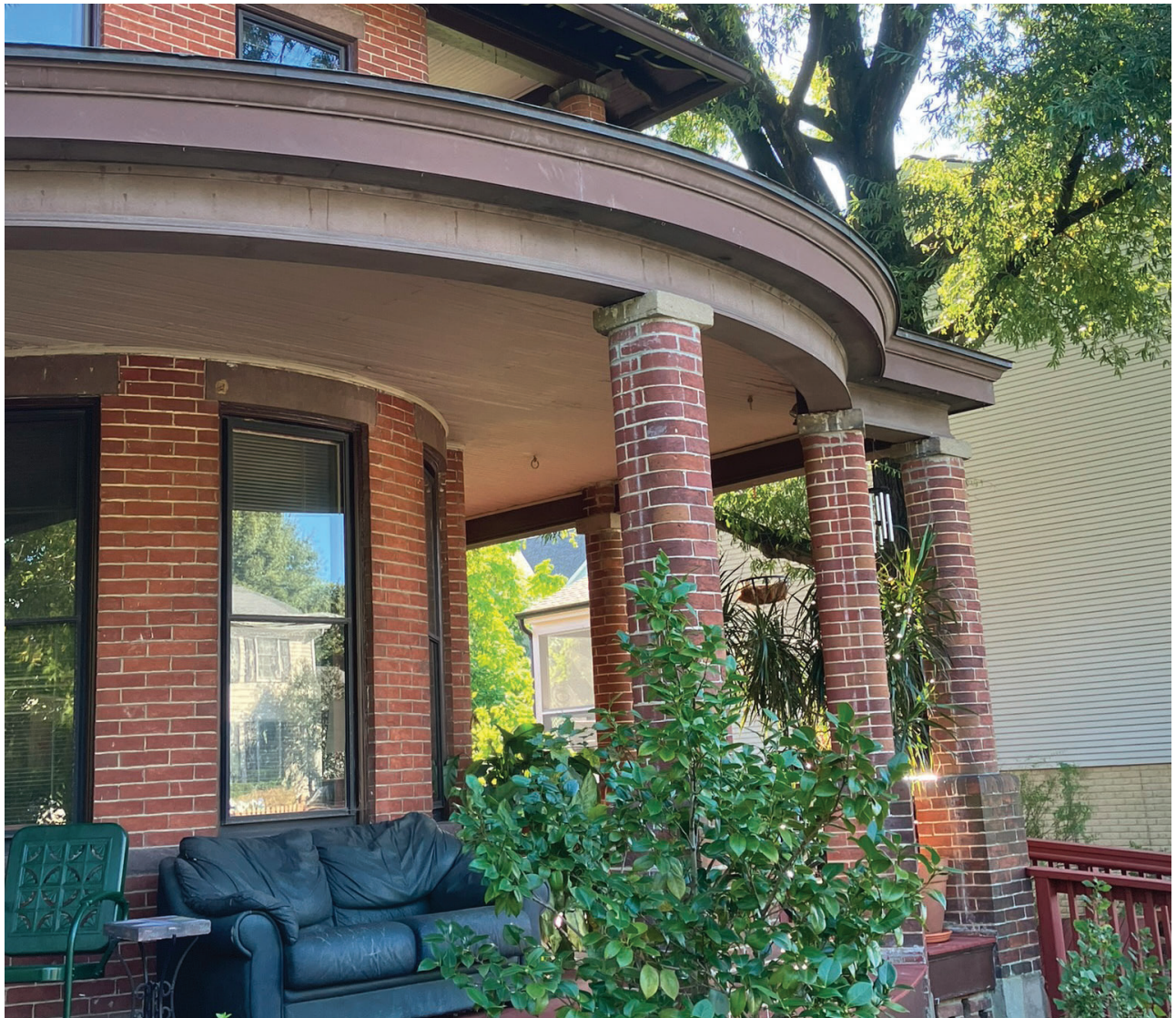
Figure 14: Detail of front porch at 3500 14th St. N. looking southwest. Source: Arlington County Historic Preservation Program, 2022.
