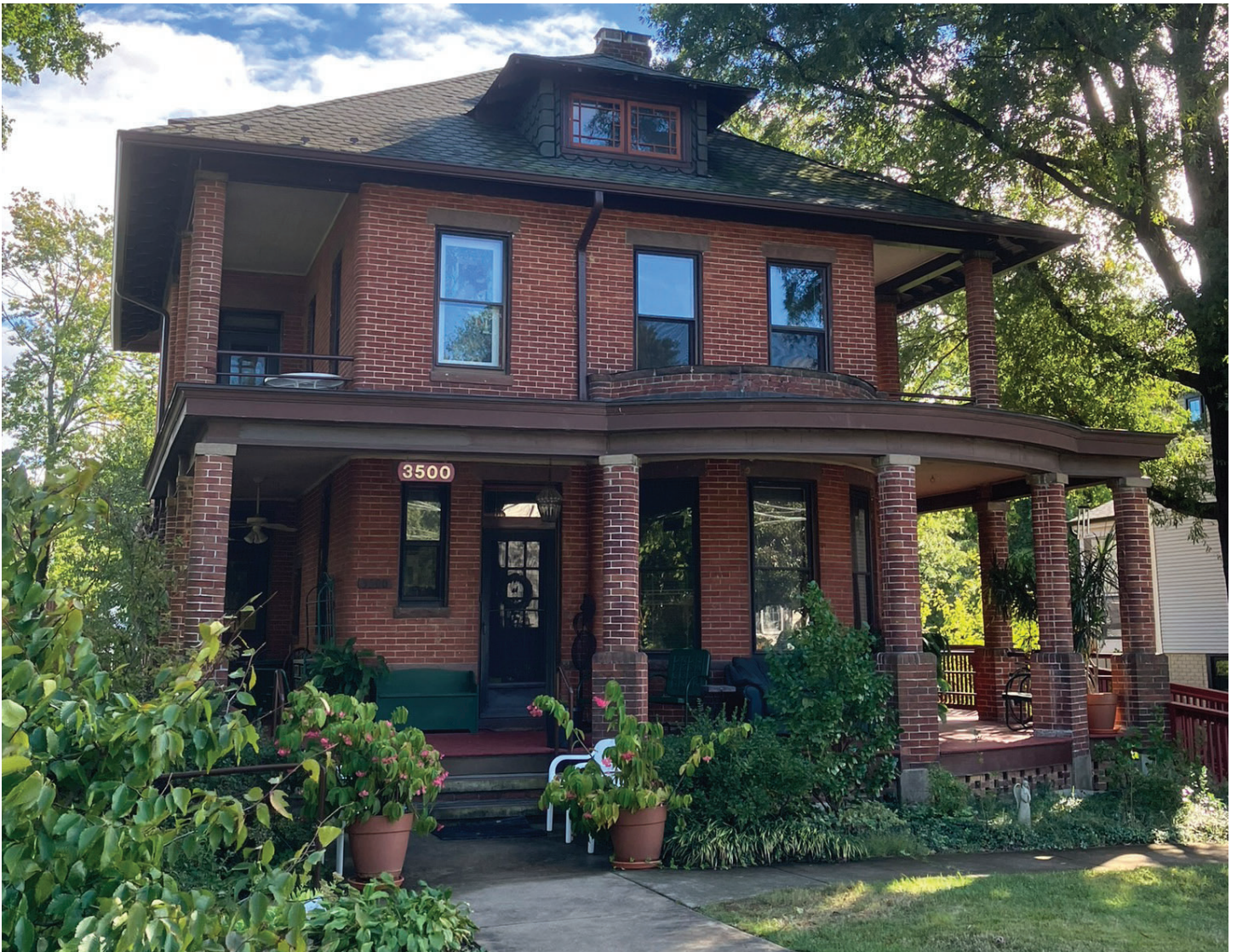
Figure 5: North facade and east elevation of the home at 3500 14th St. N. looking southwest. Source: Arlington County Historic Preservation Program, 2022.
