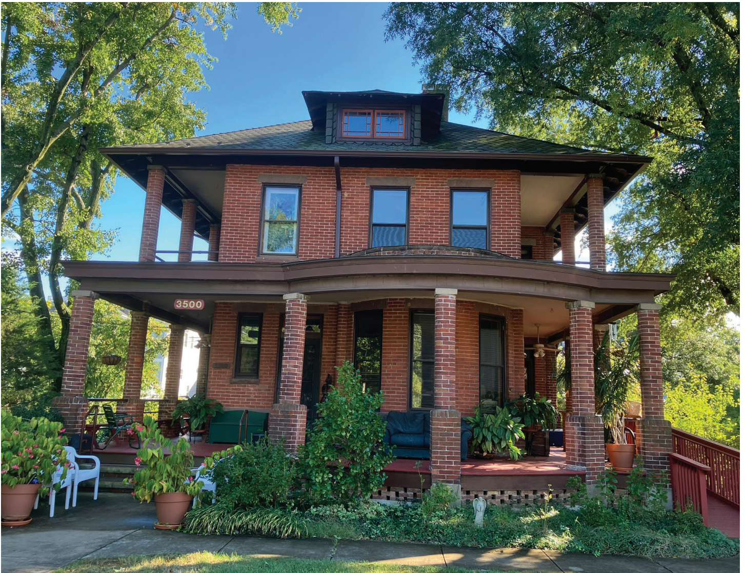
Figure 1: North facade of the home at 3500 14th St. N. looking south.
