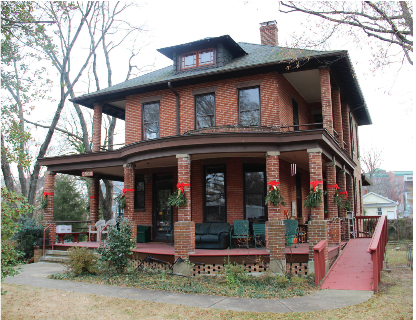
Figure 3: North facade and west elevation of the home at 3500 14th St. N. looking southeast. Source: Arlington County Historic Preservation Program, 2018.
