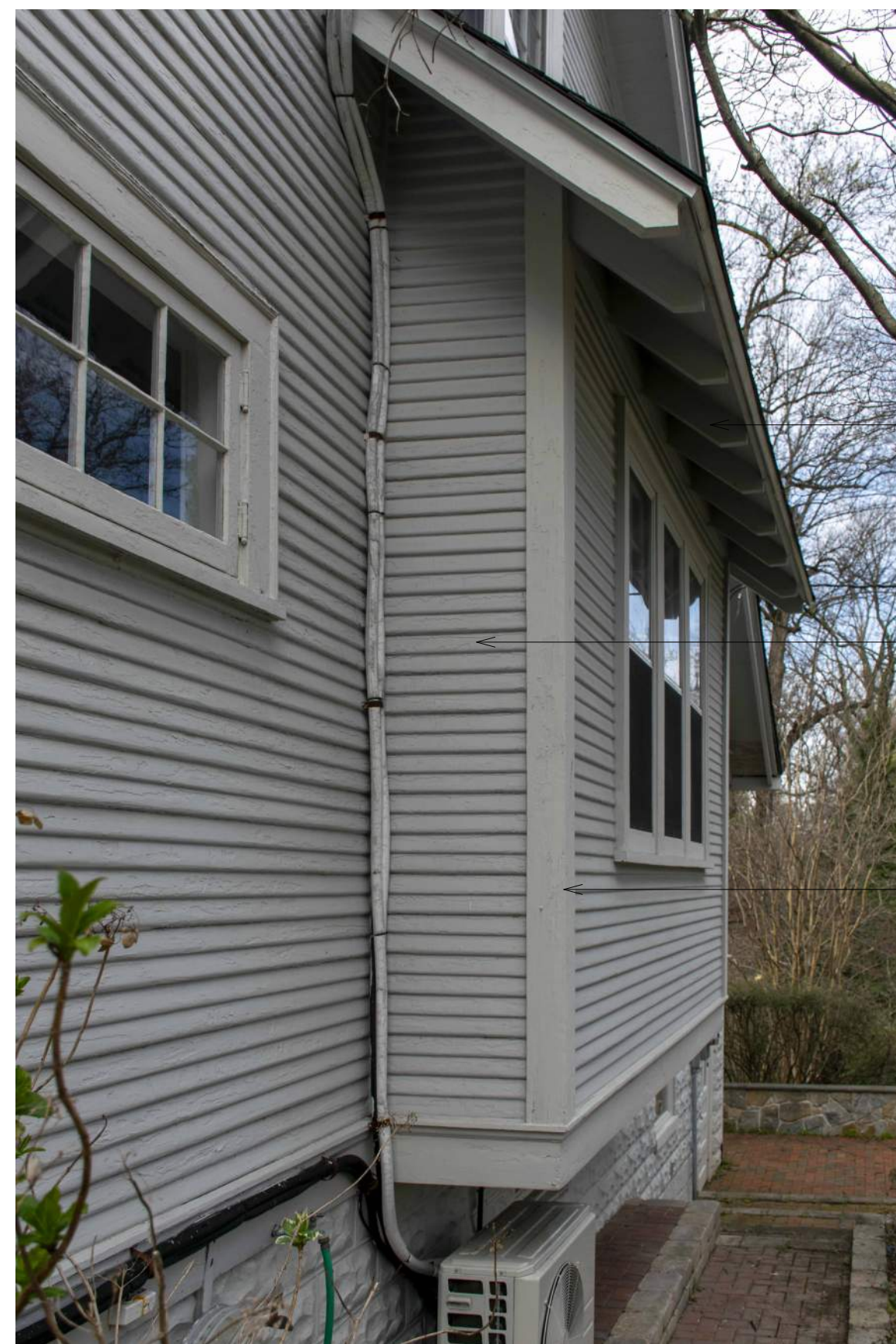
PROPOSED ROOF OVERHANGS MATCH EXPOSED RAFTER STYLE
