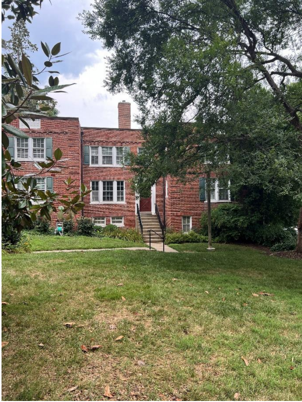
Front View from Courtyard
