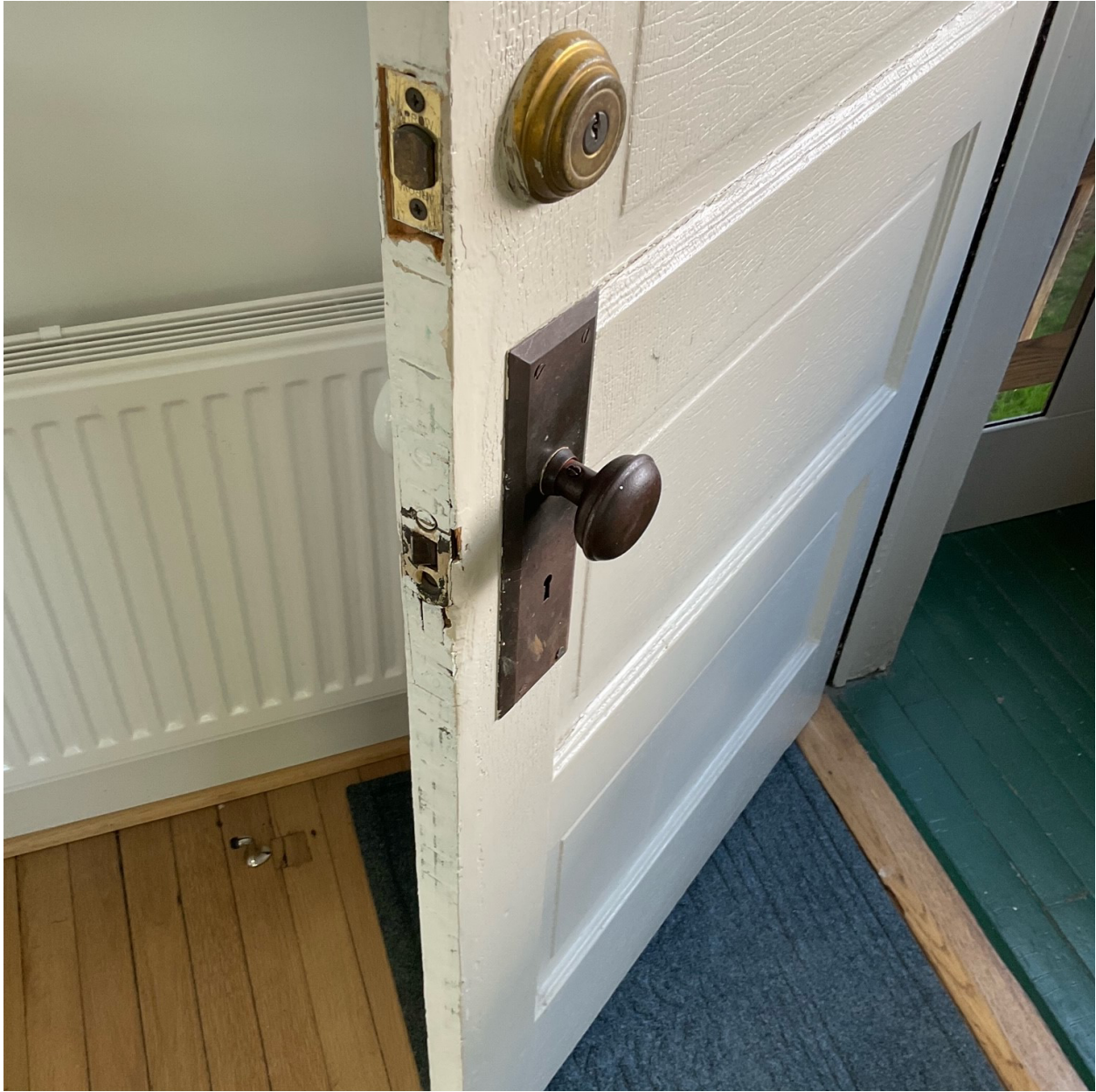
Original Kitchen door
