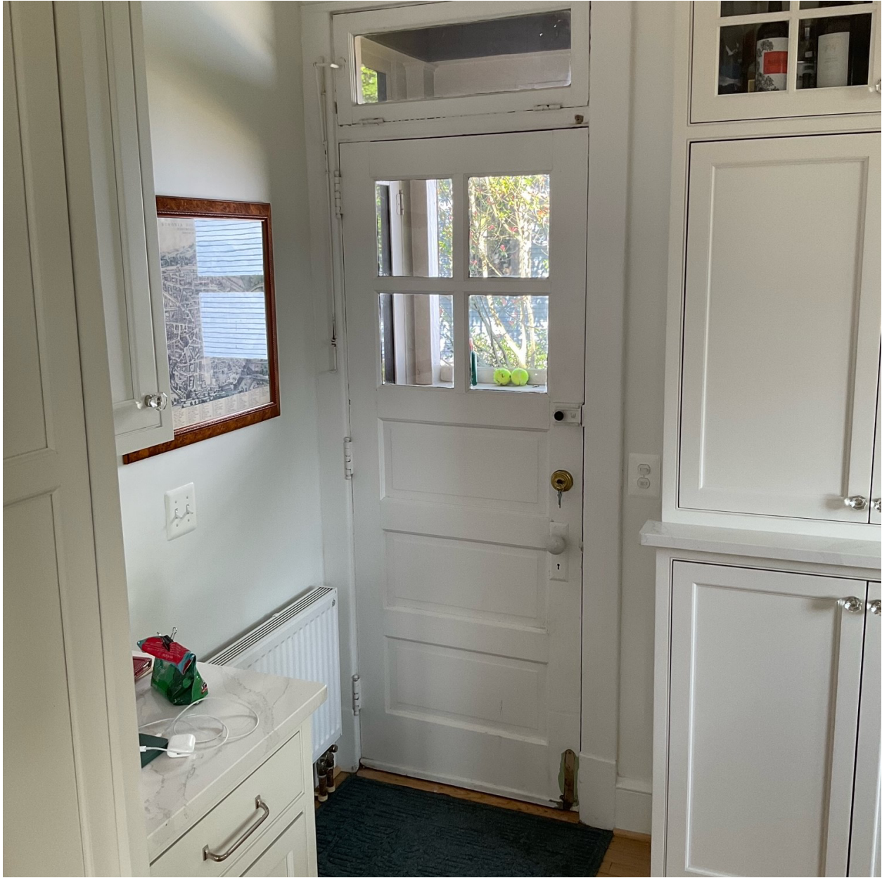
Original kitchen door
