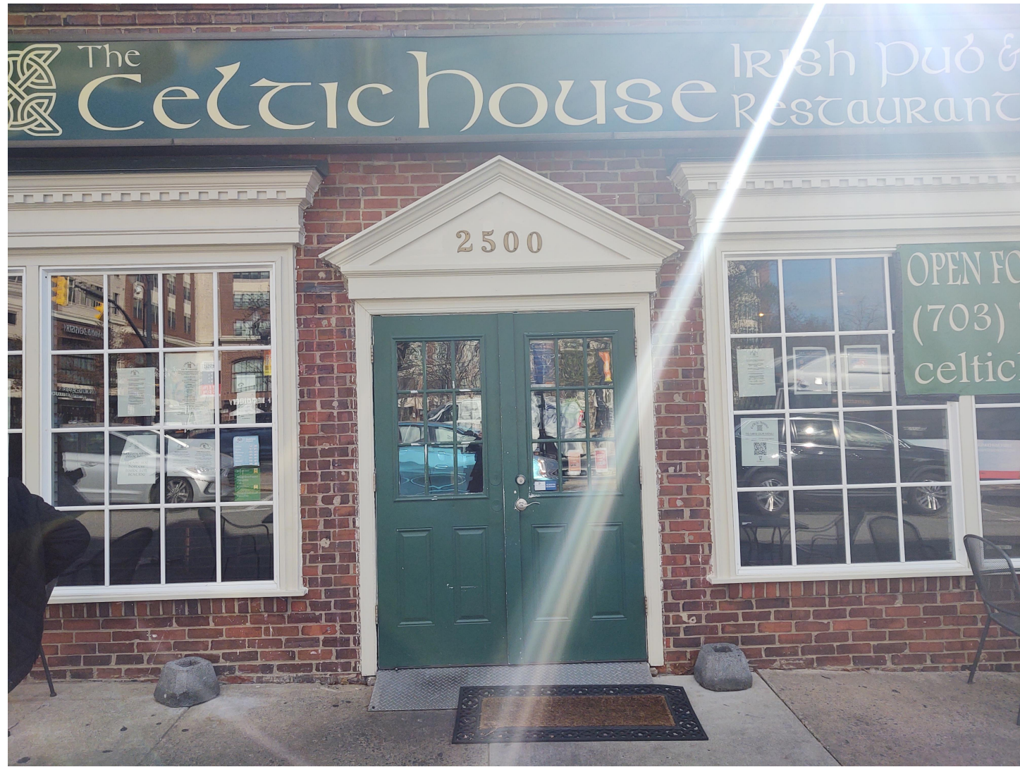
Celtic House Columbia Pike Front elevation - Entry Detail
