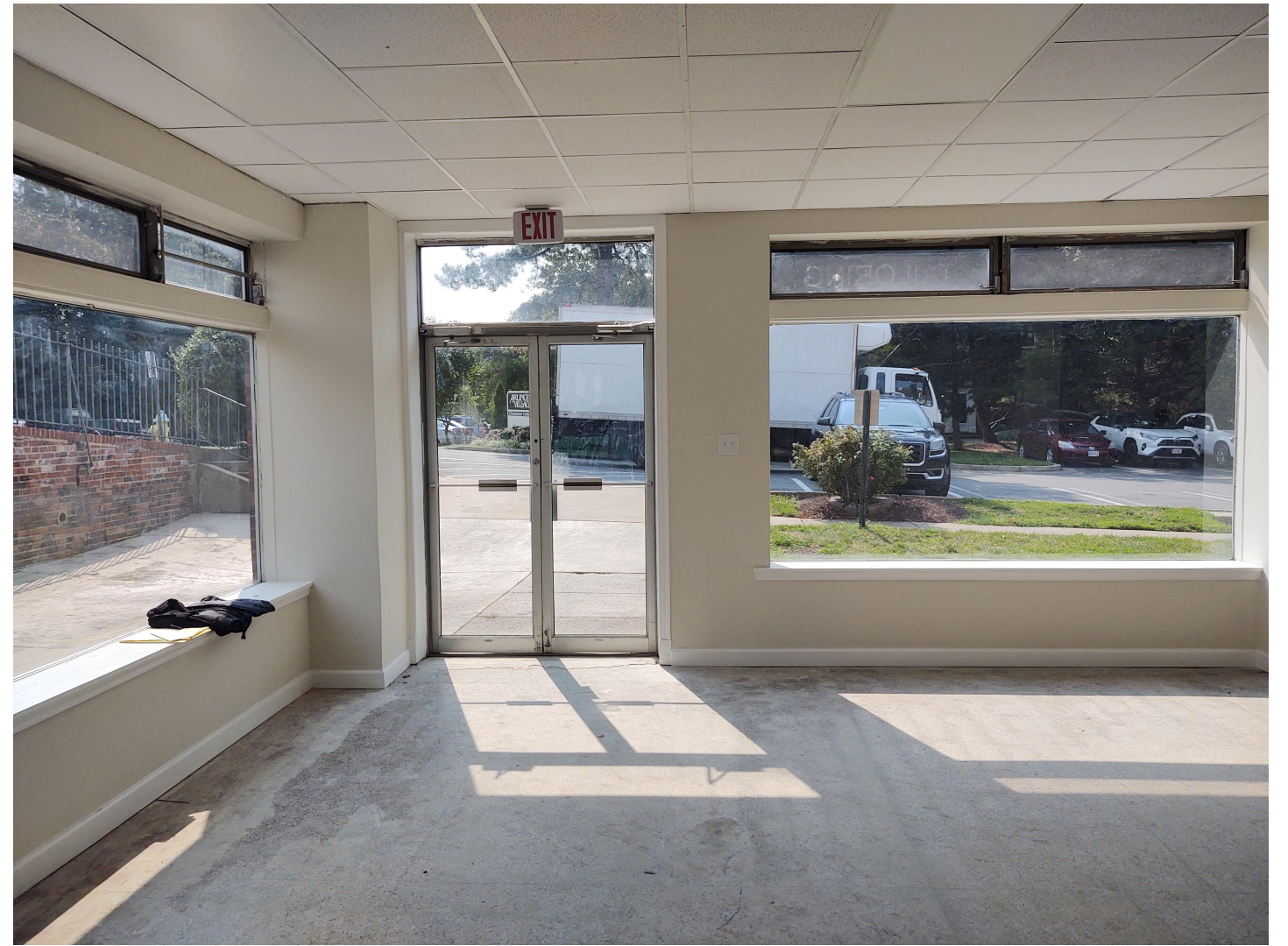
Celtic House interior of space at area of proposed work
