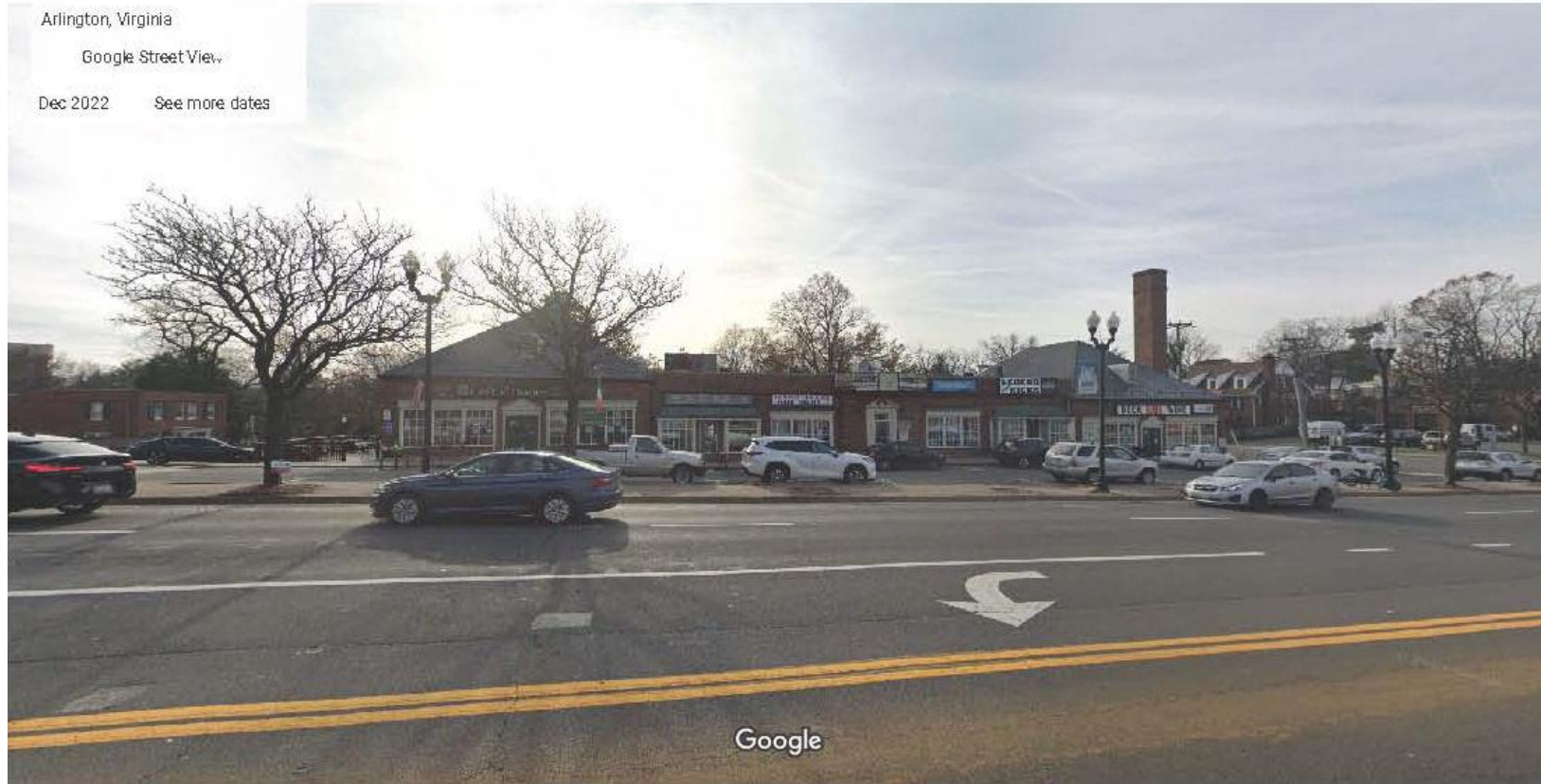
Shopping Center - Rear elevation - View of front of building
