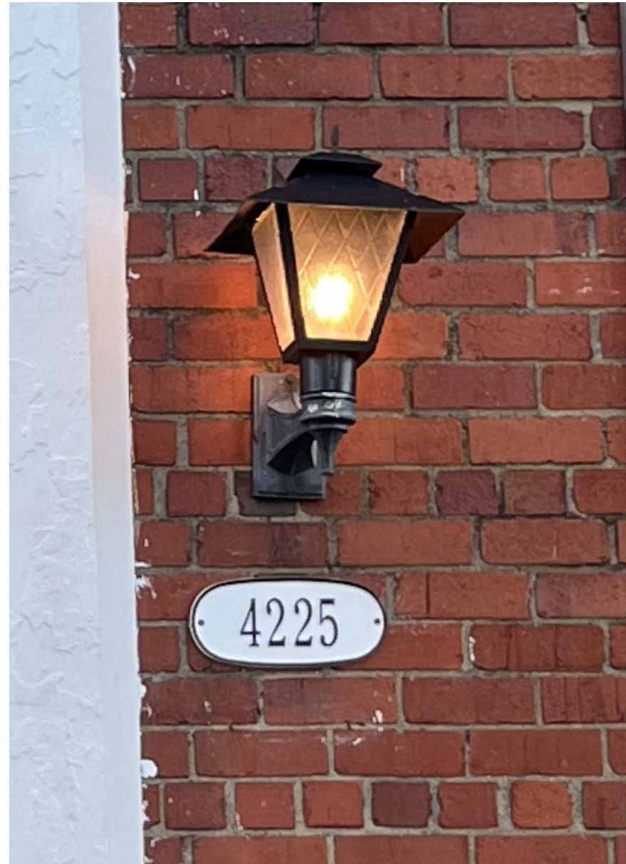
/ EXISTING LIGHT FIXTURE
