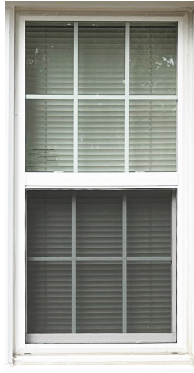
TYPICAL EXISTING WINDOWS
