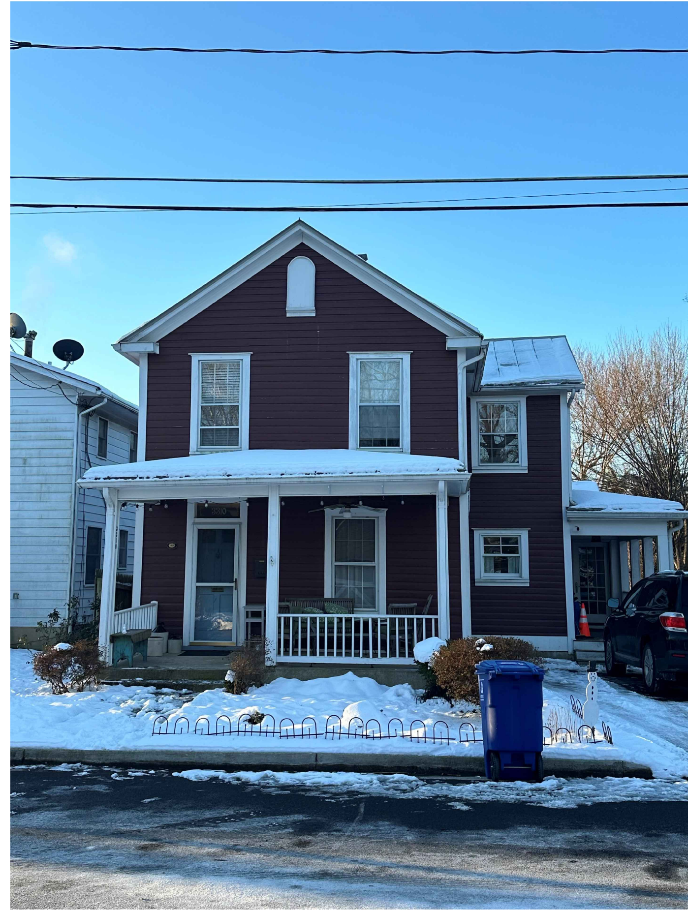
EXISTING FRONT VIEW OF MAIN HOUSE
