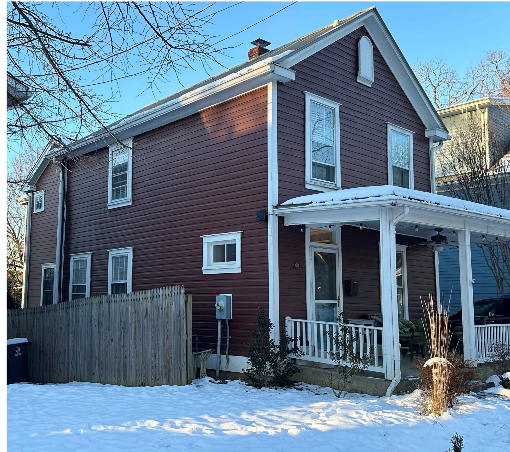
EXISTING LEFT SIDE VIEW OF MAIN HOUSE
