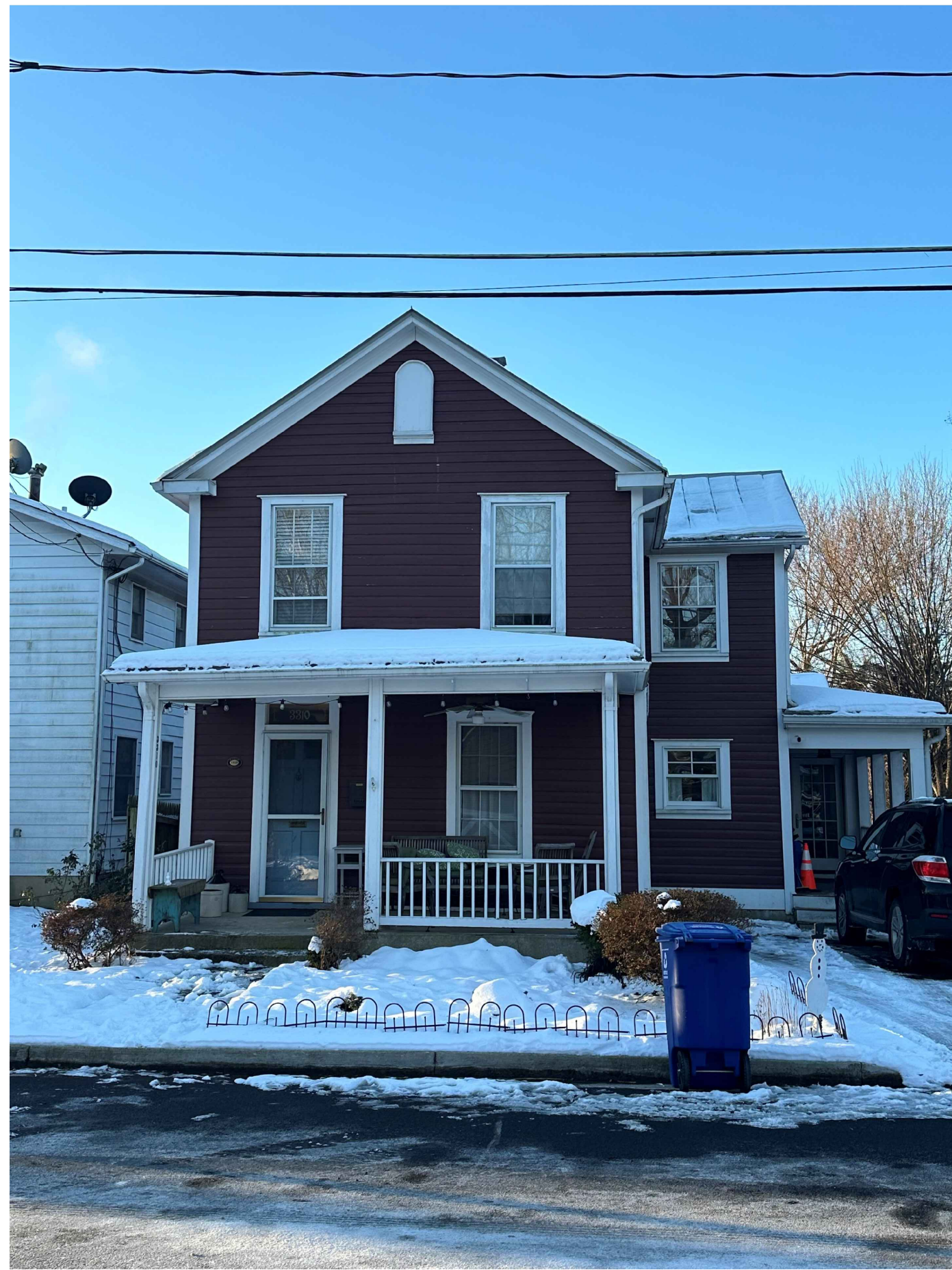
EXISTING FRONT VIEW OF MAIN HOUSE
