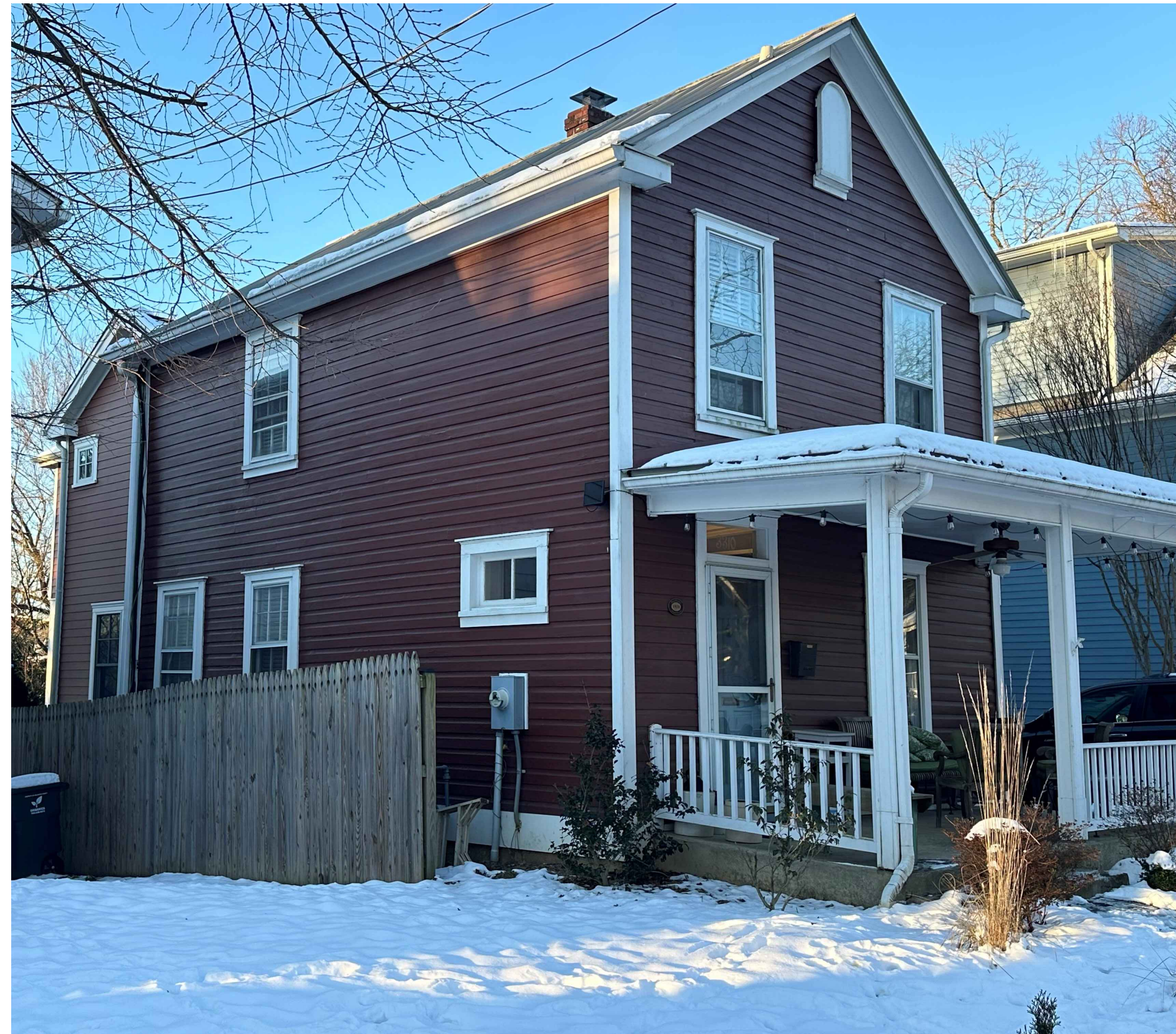
EXISTING LEFT SIDE VIEW OF MAIN HOUSE
