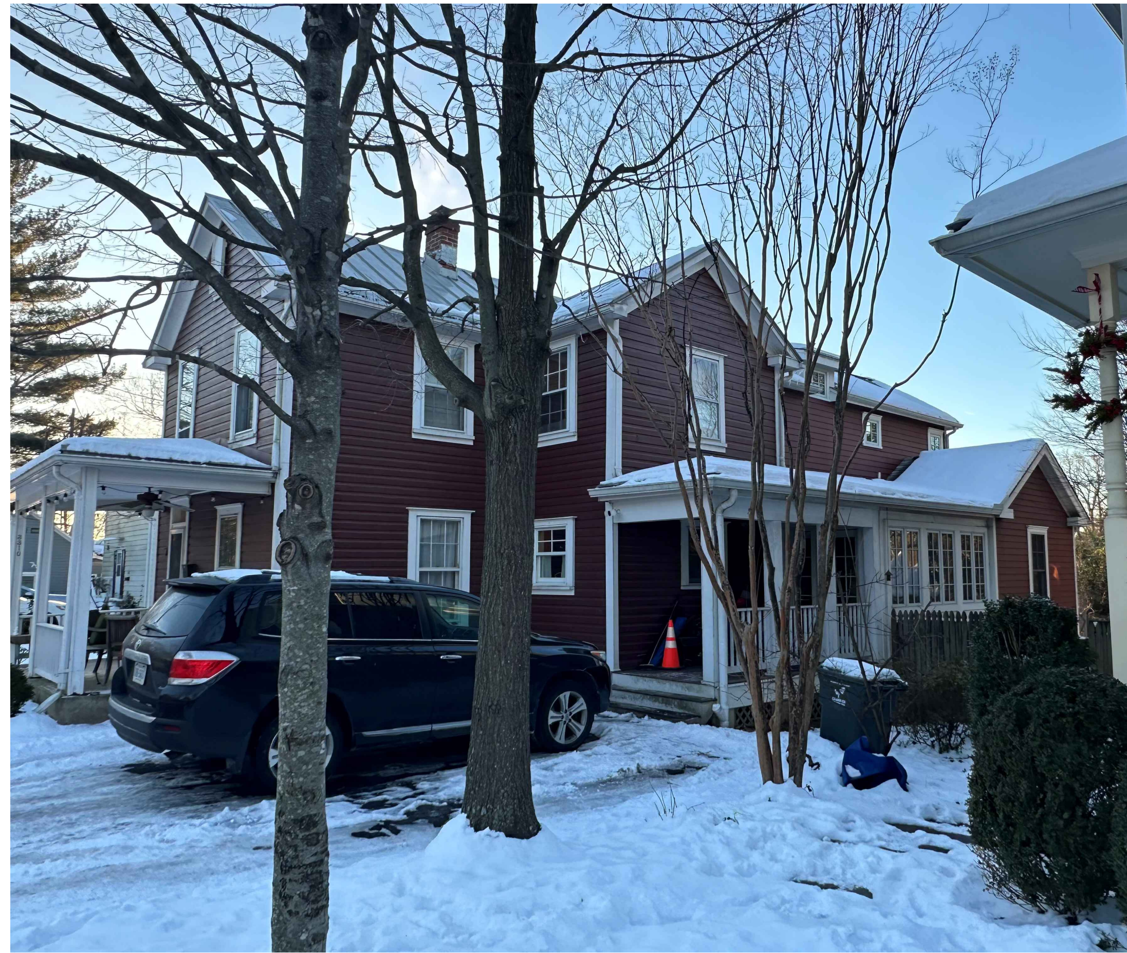
EXISTING RIGHT SIDE VIEW OF MAIN HOUSE
