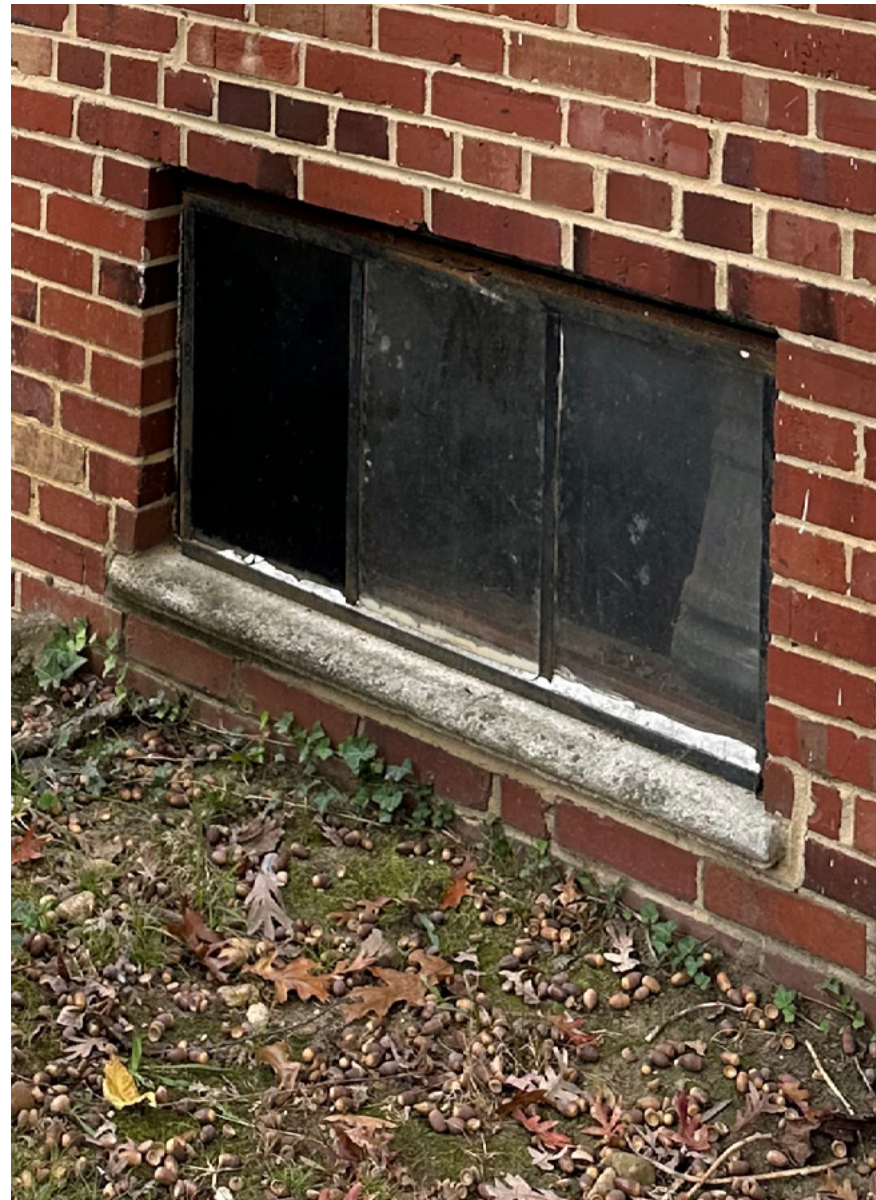
EXISTING BASEMENT WINDOW
