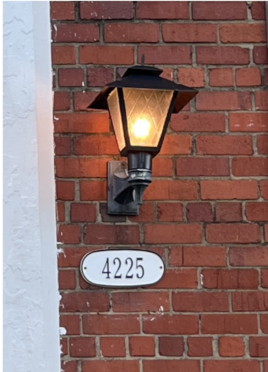
/ EXISTING LIGHT FIXTURE
